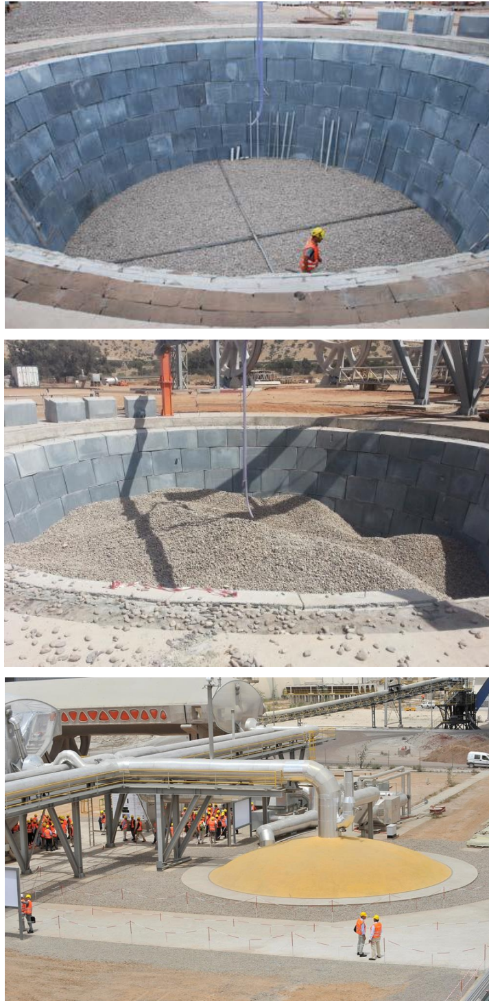
Figure 16: Pictures of the TES unit during construction: top) first layer of rocks with thermocouples sustaining structure; middle) containing tank filled with rocks, bottom) TES system completed. (Courtesy of Airlight energy SA).
