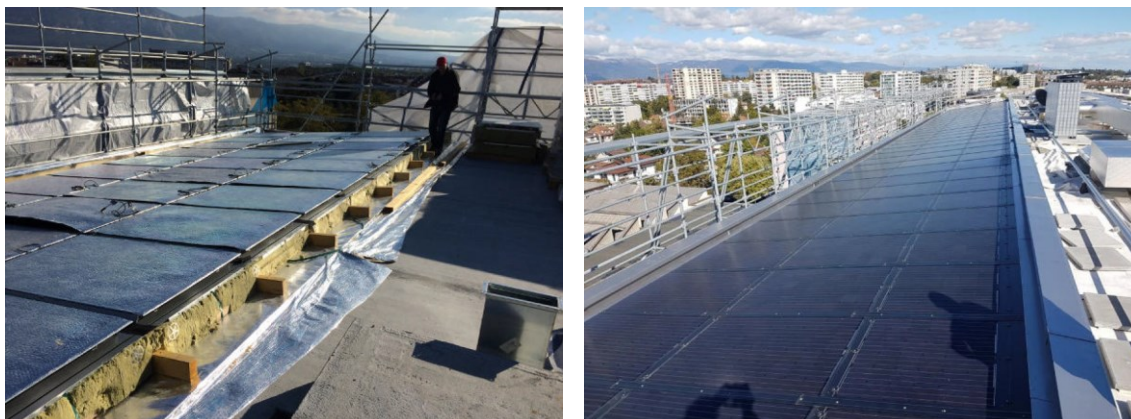
Fig. 6: Modules installés
