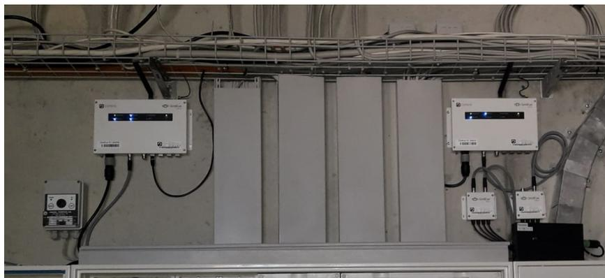
Figure 3. GridEye devices installed in Chapelle-sur-Moudon with different measurement rates of 10-min and 1-second.
