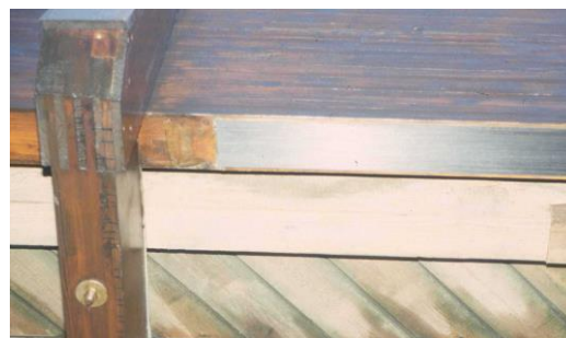
Figure 9.9. Reinforcement with CFRP laminates.
