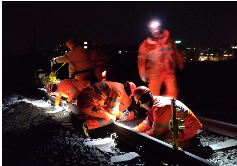
Figure 1: Installation of the Semperit railpads on 18 March 2022
