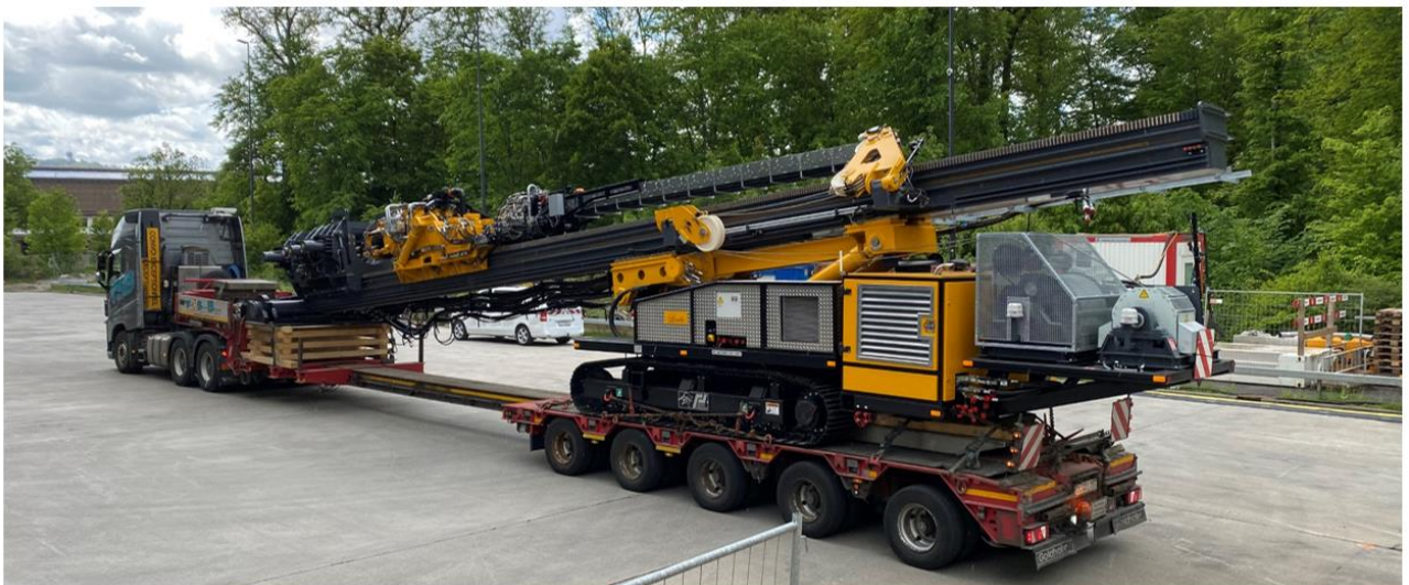
Figure 25: Delivery of rig on site.
