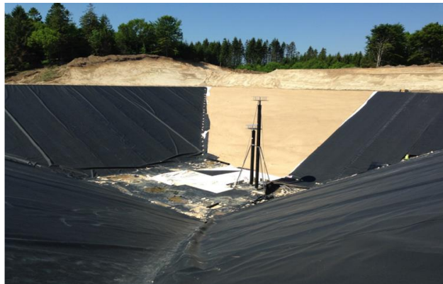
Figure 38: Picture of the inlet/outlet pipes coming from the bottom of the PTES in Dronninglund, stabilized by cables.
