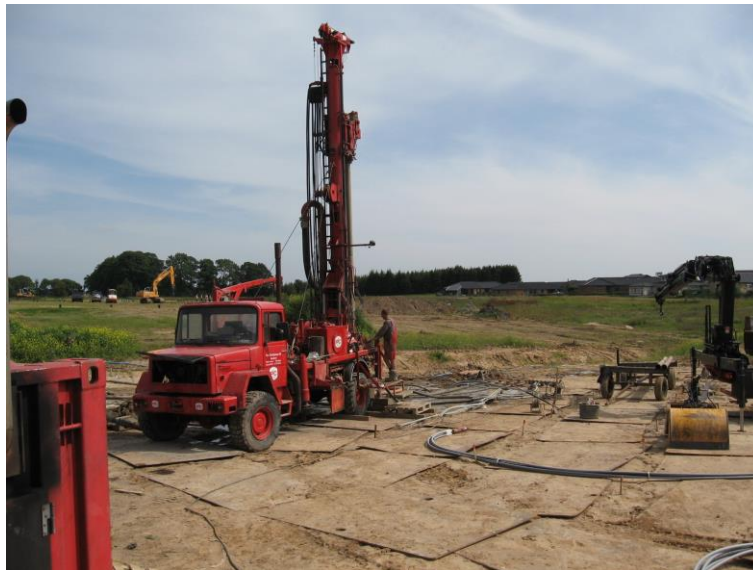
Figure 35: Picture of the wash drilling equipment used in Brædstrup.
