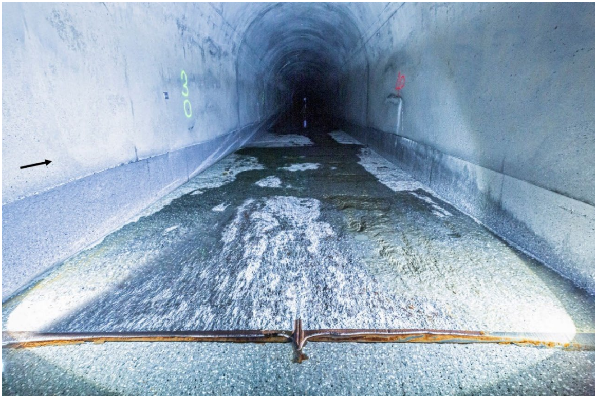
Figure 25: Picture of test field F1 (HSC) during measuring campaign of 10th December 2020 at Solis SBT, view in flow direction.
