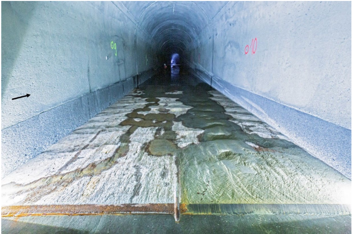
Figure 28: Picture of test field F4 (UHPC) during measuring campaign of 10th December 2020 at Solis SBT, view in flow direction.
