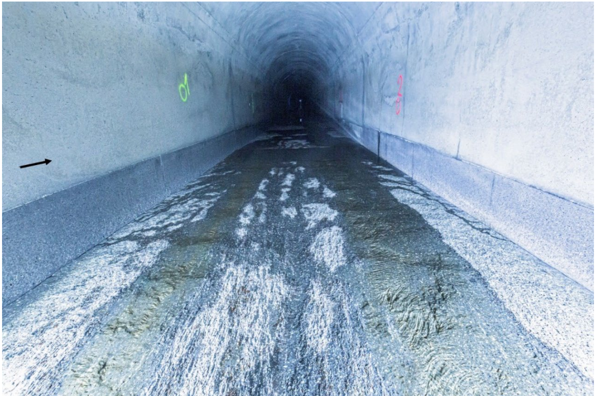
Figure 24: Picture of test field F0 (NC) during measuring campaign of 10th December 2020 at Solis SBT, view in flow direction.
