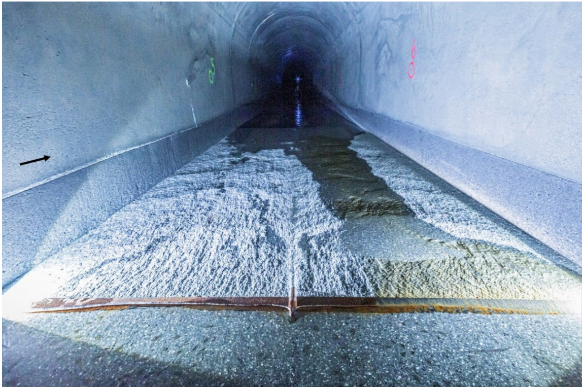
Figure 26: Picture of test field F2 (LSC) during measuring campaign of 10th December 2020 at Solis SBT, view in flow direction.
