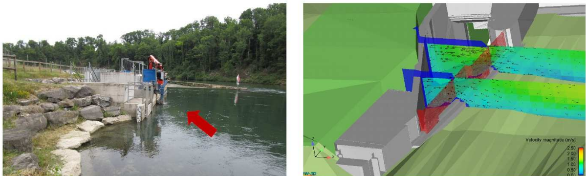
Figure 11: Horizontal Bar Rack - Bypass System-at Schiffmühle HPP: Reality (left) vs. model (right).
