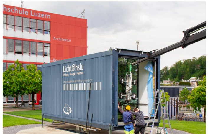
The light measurement container on the HSLU campus in Horw during the installation of the electrochromic glass. Photo: Licht@hslu
