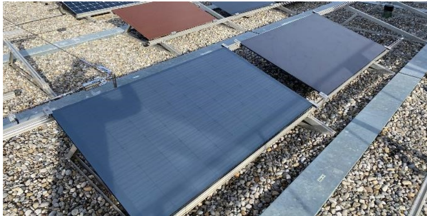
Figure 15 Image of the two-colour prototype produced by ertex and installed by CSEM on a flat roof of a building in Neuchatel (left: inkjet printing; right: screen printing)
