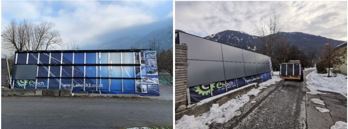
Figure 1: Prepared façade for the installation of the modules (left), completed façade installation and start of the installation of the roof system
