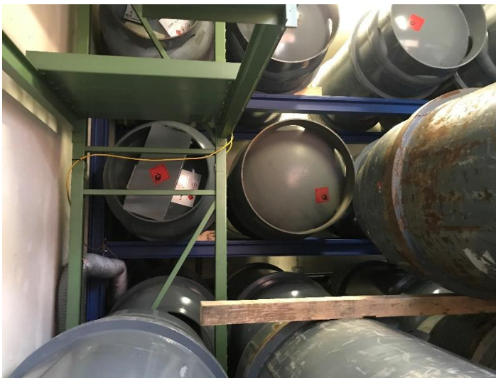
Figure 2: Storage of DME cylinders at Empa's ex-prevented storage room
