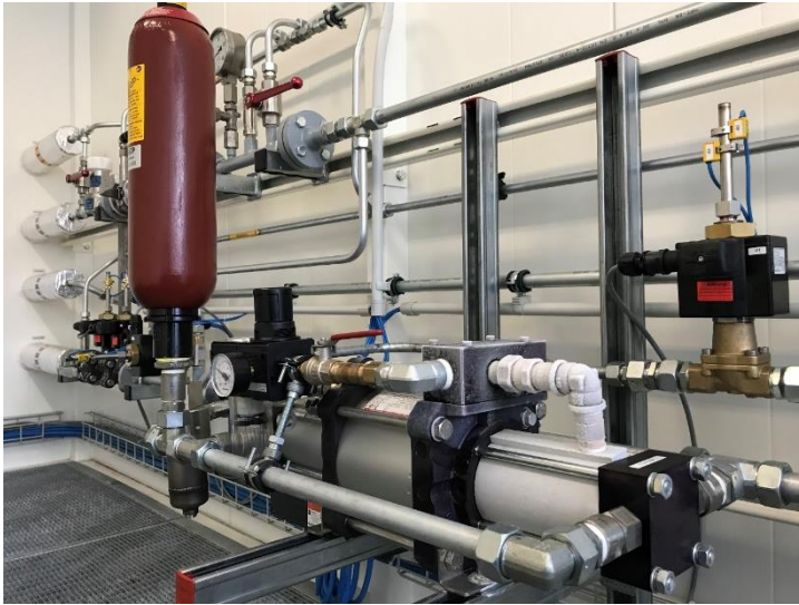
Figure 4: Pneumatic DME delivery pump plus other technical installations inside the container
