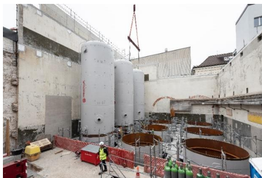
Figure 2 Storage facility for Dolderweg district heating in Basel [33]
