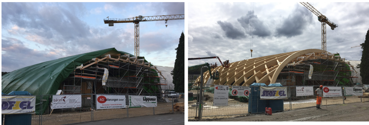
Figure 67: Efficient protection during evenings, nights and weekends or during rain; removing of the protection during the working times (Swatch building, Biel/Bienne)
