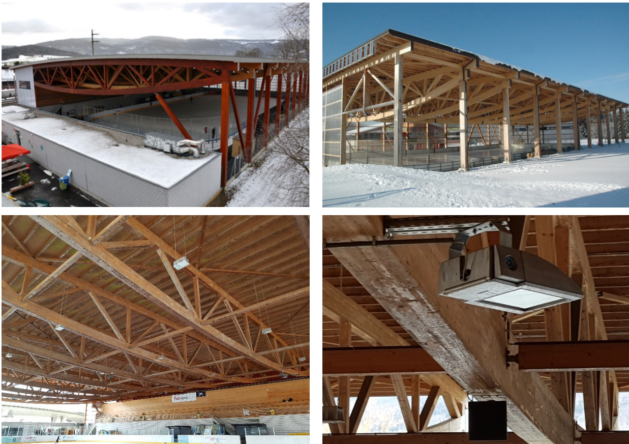
Figure 19: Pictures of the outside and inside of the ice rinks of Delémont (upper left) and Le Locle (upper right) (sources unknown) and pictures of the interiors of the Delémont ice rink with the ice formation on the downward facing surfaces of the load bearing members (bottom right)
