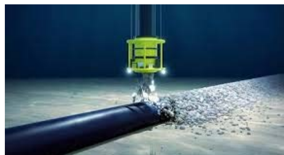
Gravel dumping for stabilization of pipe
