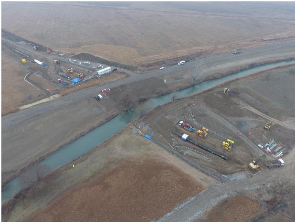
Figure 5.5.2: Trenchless installation for road crossing
