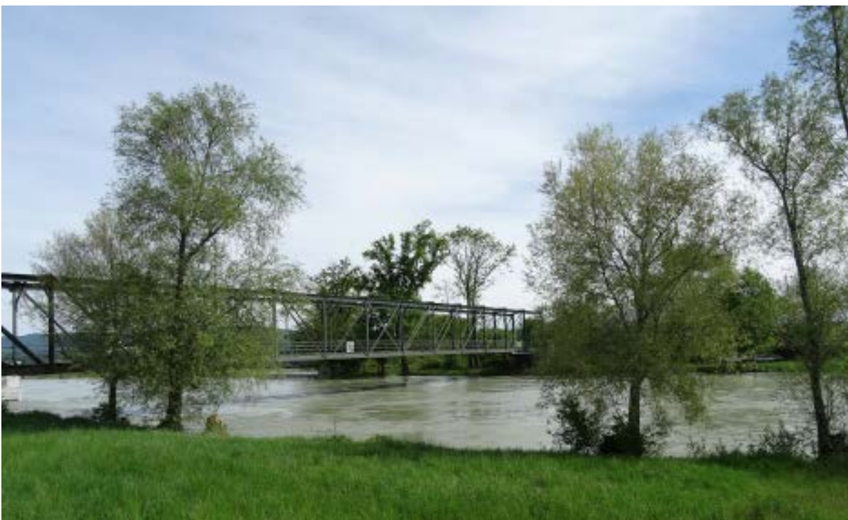
Figure 5.5.5: Aerial Bridge for an existing gas pipeline bridge parallel to CO2 pipelines routes west of Bienne
