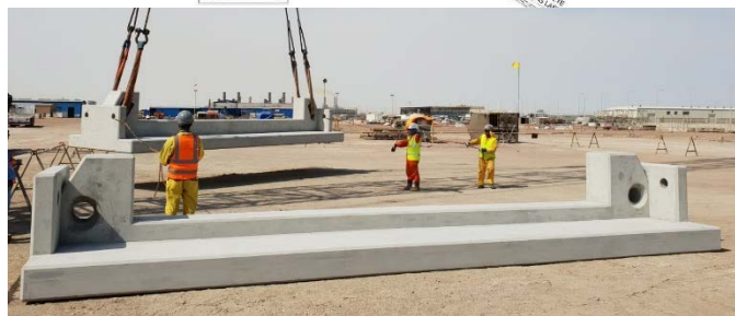
Crossing and concrete sleeper.
