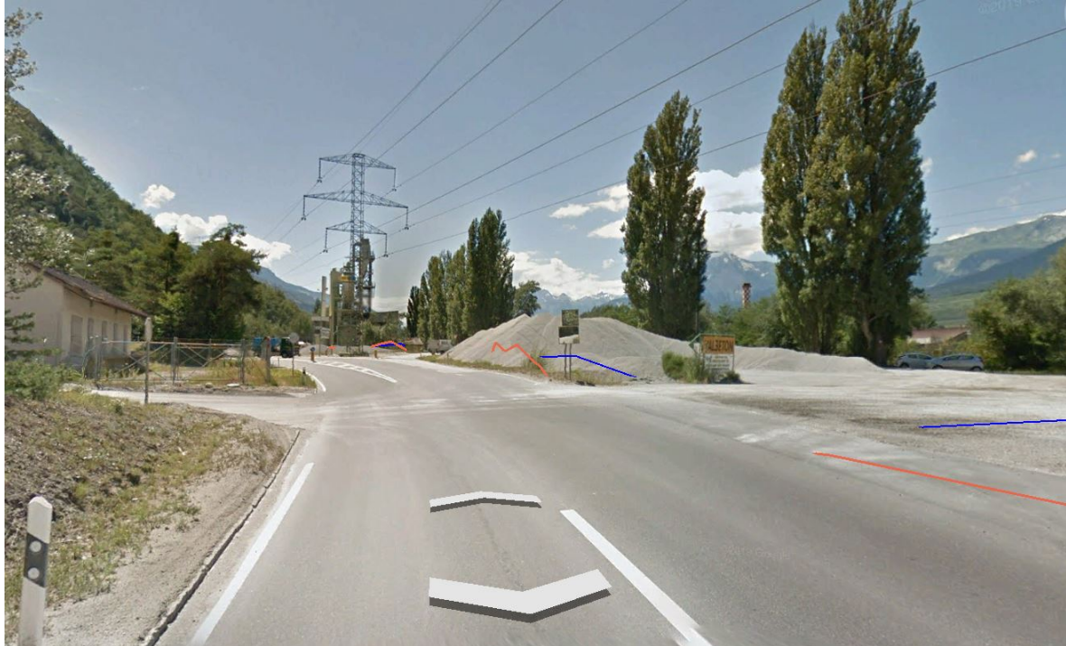
Figure 6.4.4: Lonza Flowline along Rhone valley in congested situation with parallel gas pipeline
