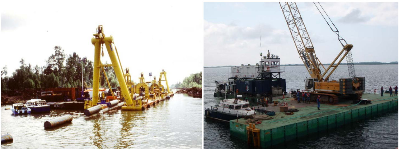
Laybarge and crane barge assembled with Combifloat moduli
