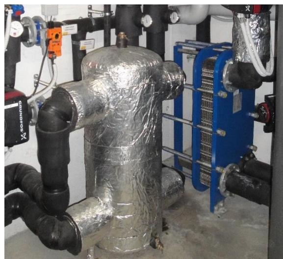
Figure 6 – Hydraulic separator (insulated to prevent condensing).
