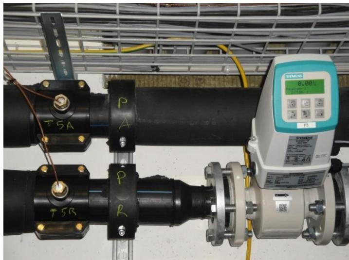
Figure 5 – Heat meter, with 1 flowmeter (on the right) and 2 thermocouples (on the left).
