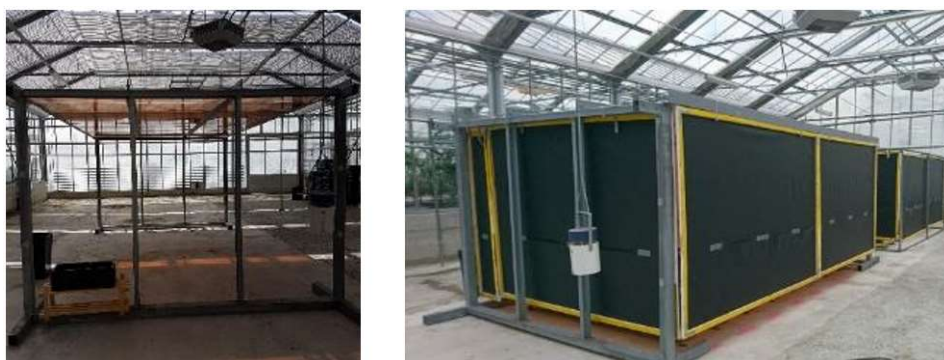
Figure 4: Stages of greenhouse preparation. Bottom left: the DSC pod before cladding. Right: Both 15 m 2 greenhouse test enclosure with DSC modules and without DSC modules.
