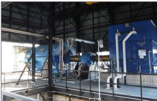
Figure 15: Examples of LP-compressor (left picture) and HP-compressor (right picture) suitable for the AA-CAES charging process
