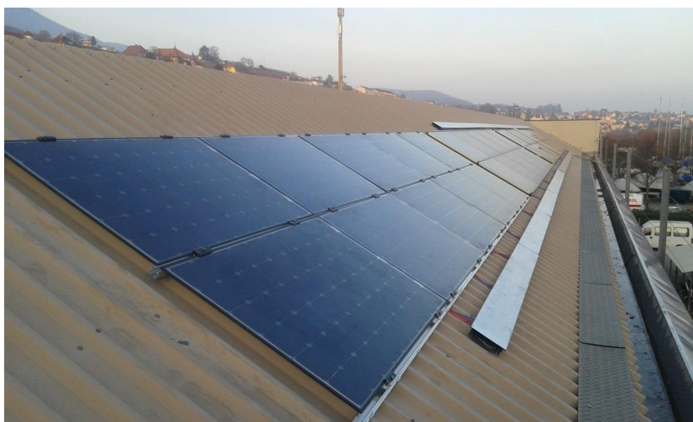
Figure 1.23: outdoor installation of 40 module, 10 reference and 30 modules produced within the Swiss Inno-HJT project
