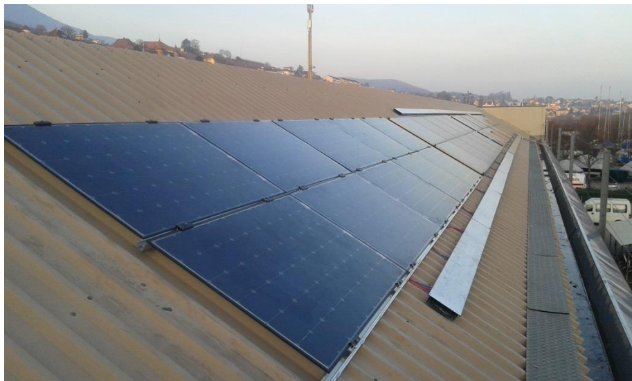
Figure 3.2: Four 3 kWp demonstration systems installed on the Innoparc building in Hauterive (NE). In the foreground are frameless Gen 2 and Gen 3 modules connected in November 2016.
