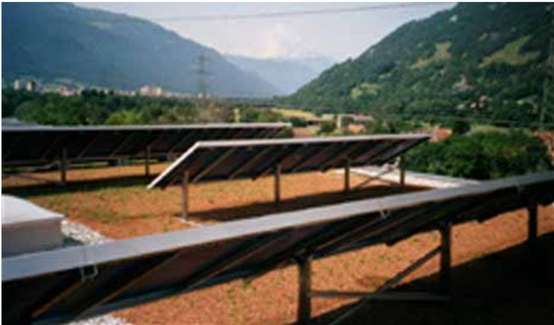
PV array on a flat green roof, in Chur (Switzerland), 10 kW, 2000
