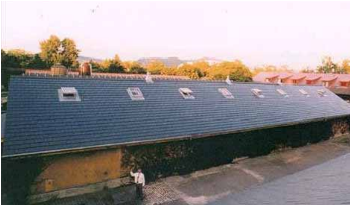
Photovoltaic roof in Bern (Switzerland), 92 kW, 1998, built by Atlantis Solar Systems (Bern, Switzerland)
