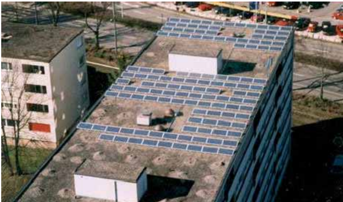
Private residential of Mr. Hafner (Hirzenbachstr.)-Edisun AG in Zurich (Switzerland), 12.6 kW, 1998, built by Edisun AG (Zurich, Switzerland) with Sofrel 95-20o and Shell modules
