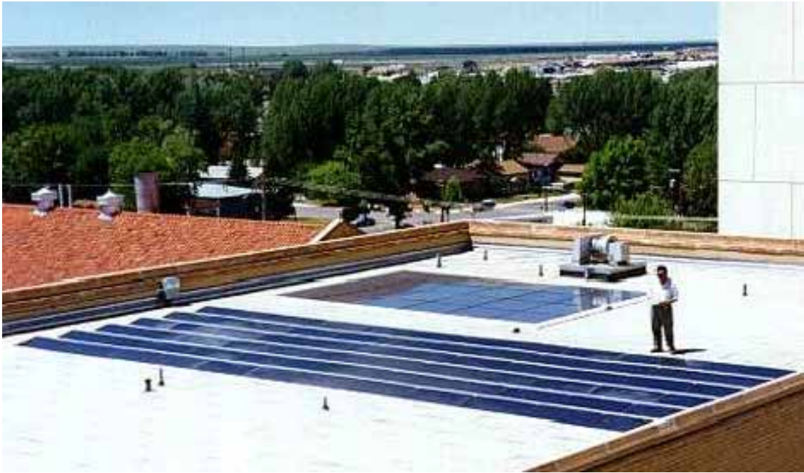
University of Wyoming at Laramie, USA, 10 kWp includes both sloped and flat tiles, 1996, built by Powerlight
