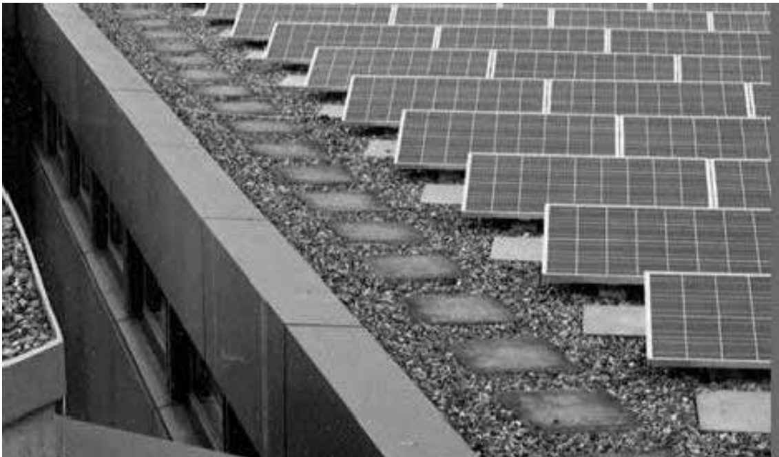
Office building in Wattwil (Switzerland), 30 kW, 1996 built by Tritec (Allschwil, Switzerland) with Sofrel 95-200 and Kyocera modules
