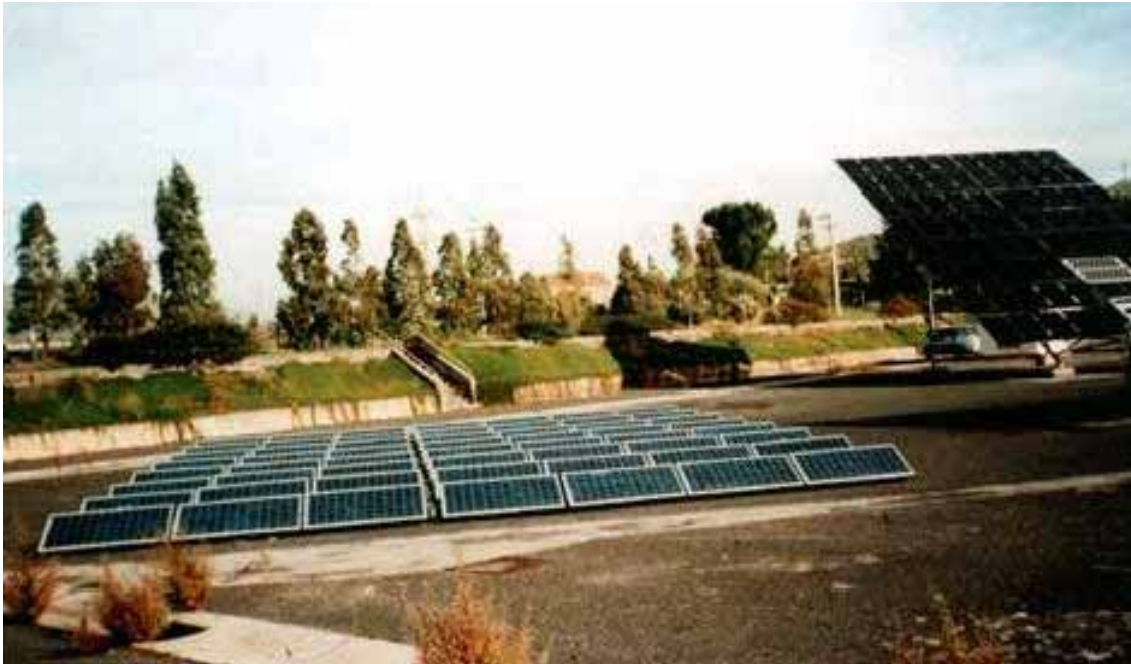
Ground based system on a test field in Adrano Sicily (Italy), 5.6 kW, 1994, built by Conphoebus and installed by ENEL.
