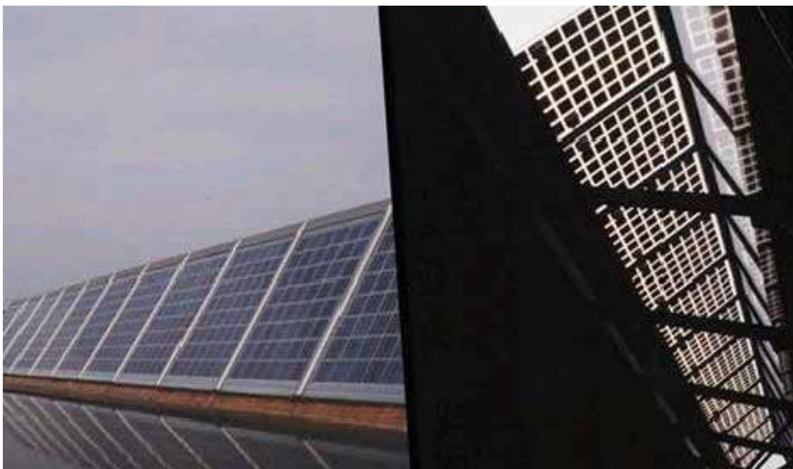
Sheds at the Swiss Federal Institute of Technology in Lausanne (Switzerland), 1.4 kW, 1994, built by Solution (Härkingen, Switzerland).
