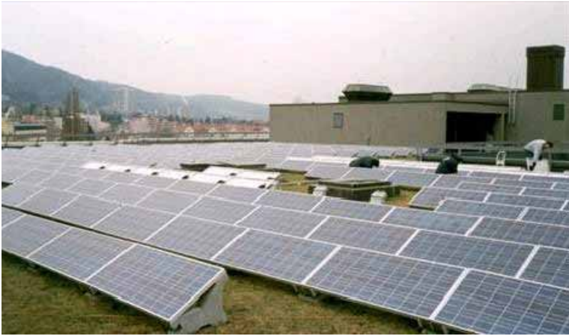
Green roof building Vita-Edisun AG in Zurich (Switzerland), 50 kW, 1998, built by Tritec (Allschwil, Switzerland) with Sofrel 98 and Kyocera modules
