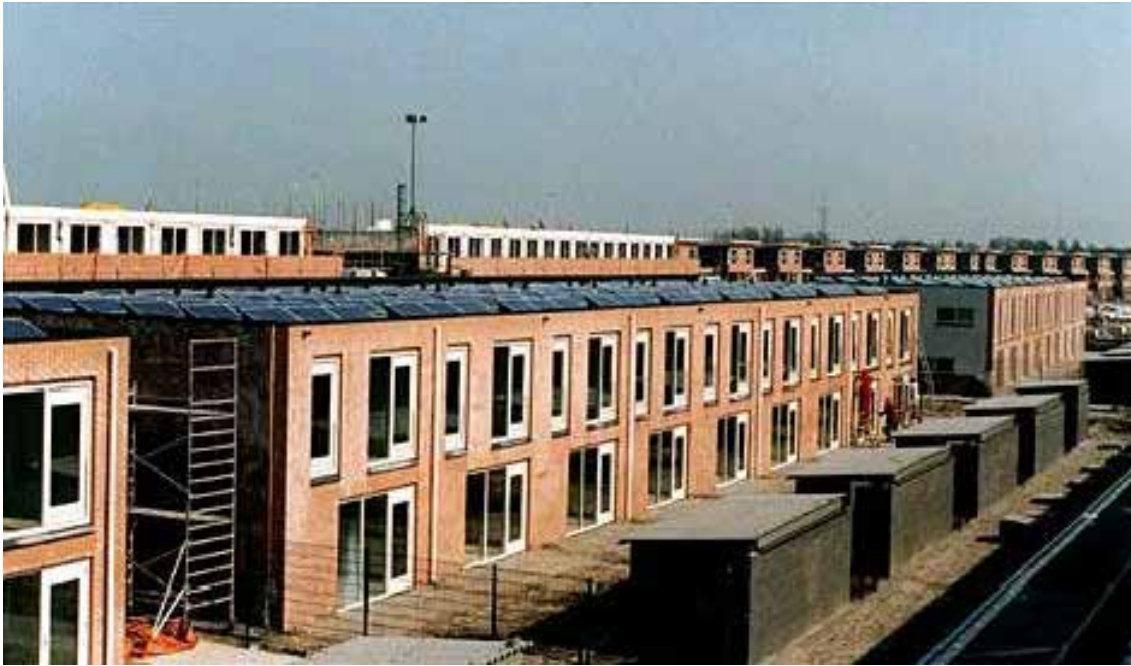
Flat roof installation in Nieuwland, Amersfoort (The Netherlands) 20 kW, 1996, installed by Ecotec (Rotterdam, The Netherlands).
