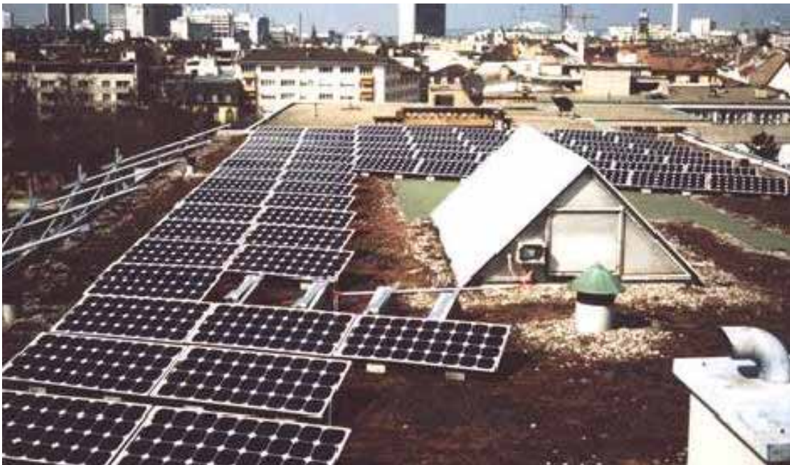
Research institute in Basel (Switzerland), 20 kW, 1996, built by Holinger (Liestal, Switzerland) with Sofrel 95-20o and BP modules
