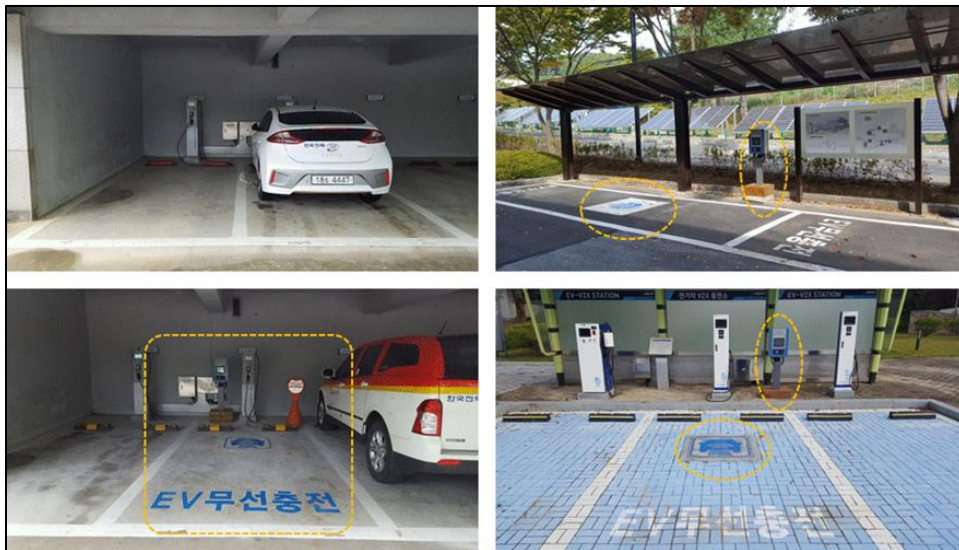
Figure 18. KEPCO and Green Power Co. installed a 6.6 kW WPT EV charging infrastructure (ground adapter) at parking lots of KEPCO Research Institute (ground surface with concrete, asphalt, blocks).
