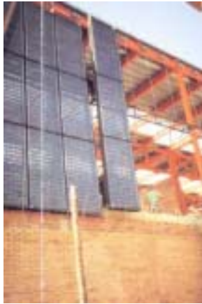
Abbildung 6: Intelligent building design and construction process - Mounting and integration of solar modules into the Mataró library building in Barcelona, Spain. The photovoltaic modules are at the same time façade elements and are part of the solar power station (53 kWp). Source: TFM, Spain.
