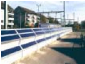
Abbildung 8: Multifunctional use of infrastructure elements - Railway noise barriers in Oerlikon-Zurich, Switzerland. Source: TNC Consulting AG-Erlenbach, Switzerland
