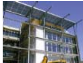
Abbildung 9: Progressive design - Mobile entrance roof with semitransparent PV modules on the "Harmony" building in the City of Tomorrow. Source: Bo01, Malmö, Sweden
