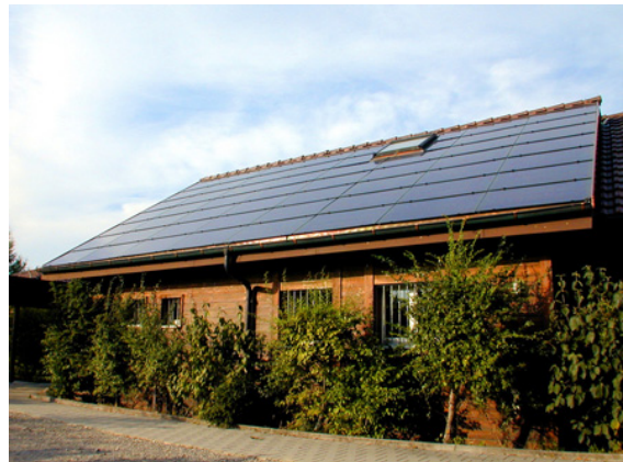
Figure 22: Pfadiheim Weiermatt roof integration installation in Köniz (Photo: NET)
