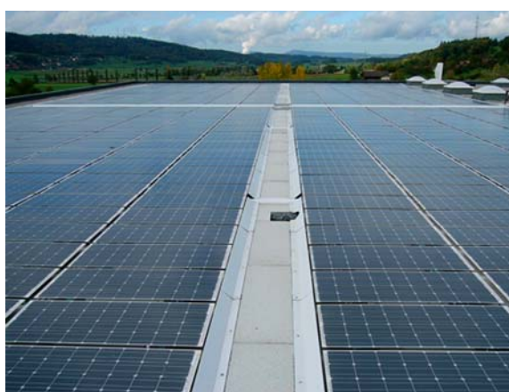
Figure 14: 62 kWp installation with PowerGuard (Photo: Zagsolar)
