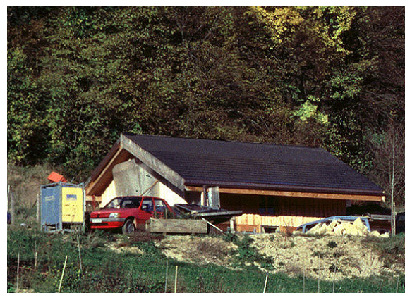
Figure 26: Stand-alone 3 kWp roof integration in Soyhières (Photo: NET)
