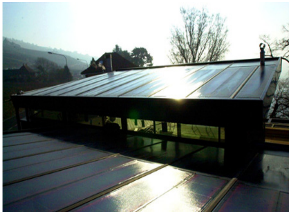
Figure 21: Freestyle® roof integration (Photo: Solstis)
