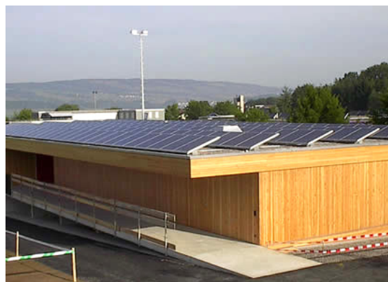
Figur 16: Hünenberg 27 kWp Alustand installation (Photo: Urs Bühler Energy Systems)
