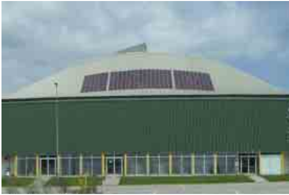
Figur 11: 2 kWp Flexcell Experimentaldach (Bildquelle: VHF Technologies)
