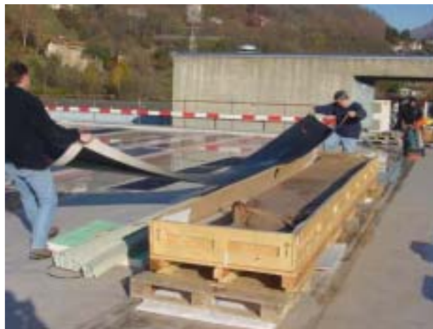
Figure 1: roofing membranes joined by mean of hot air welding.
