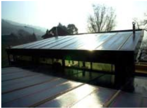
Figur 15: 5.5 kWp Dachintegration Freestyle (Bildquelle Solstis)
