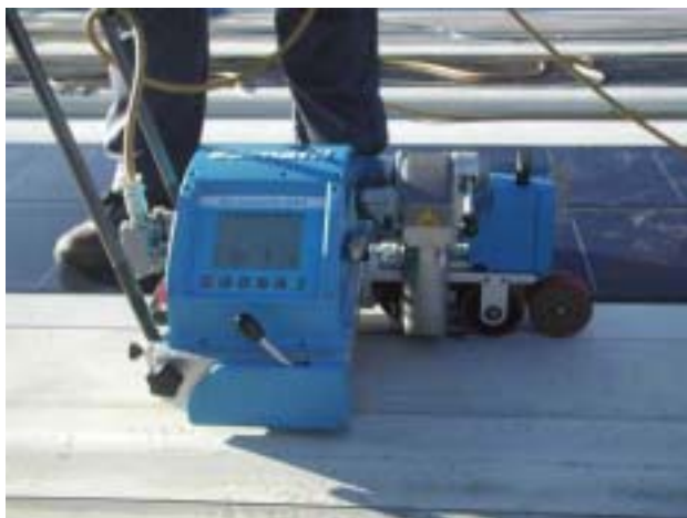
Figure 1: roofing membranes joined by mean of hot air welding.
