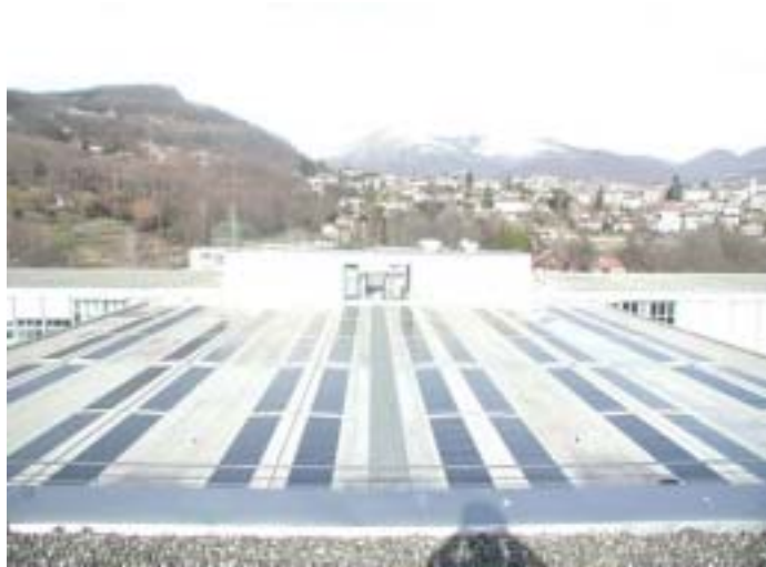
Figure 3: Flat roof integrated 15.36kWp a-Si triple-junction PV power plant.
