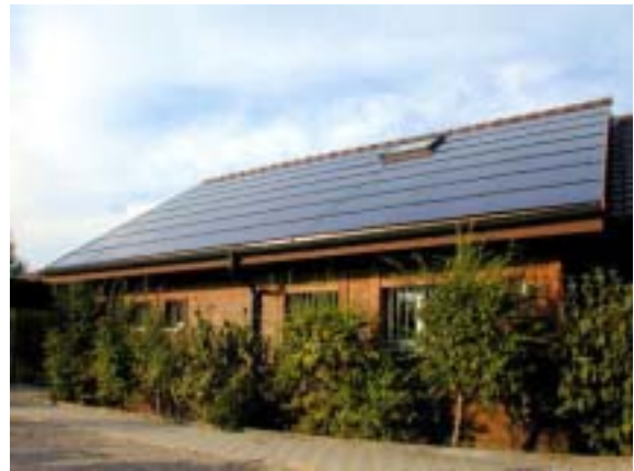
Figur 16: 15 kWp Dachintegration Weiermatt (Bildquelle NET)
