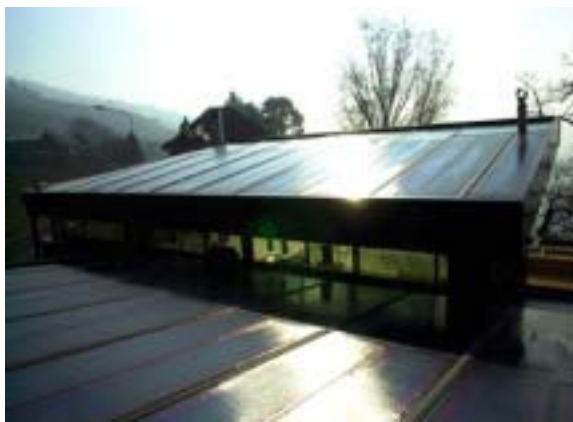
Figur 21: 5.5 kWp Dachintegration Freestyle (Bildquelle Solstis)
