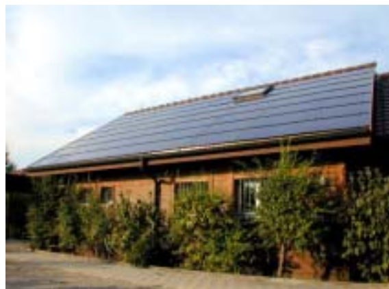
Figur 22: 15 kWp Dachintegration Weiermatt (Bildquelle NET)
