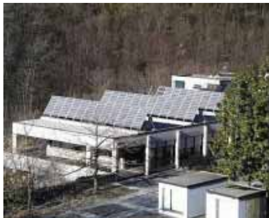
Picture 1: 10 kW m-Si PV plant
