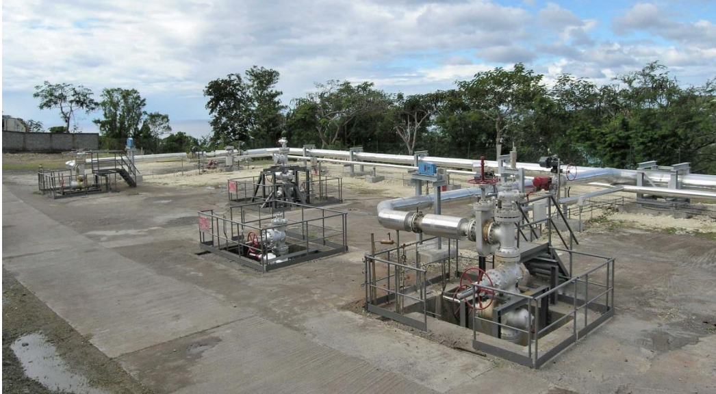
Figure 10.1 View of BO-5 and BO-6 production wells of the Bouillante geothermal plant (Guadeloupe, West Indies): the production line has been adapted at the very end of 2010 and reinforced to resist to major seismic events.
