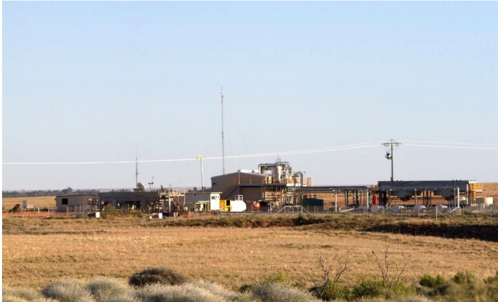
The Geodynamics Habanero 1 MW EGS power station (centre), with station air coolers (right) and brine air coolers (left), Cooper Basin, South Australia. (Photo courtesy of Geodynamics Limited)
