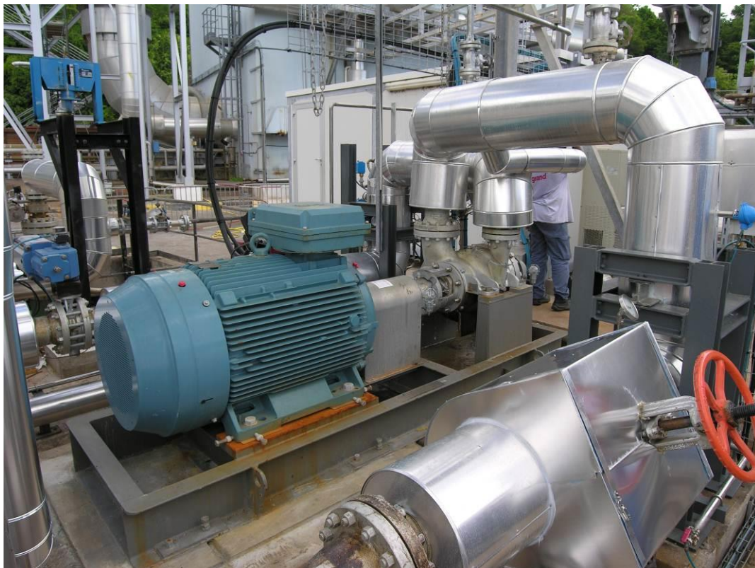
Figure 10.4 View of Bouillante reinjection: a partial reinjection has been put in place to maintain the pressure in the reservoir.
