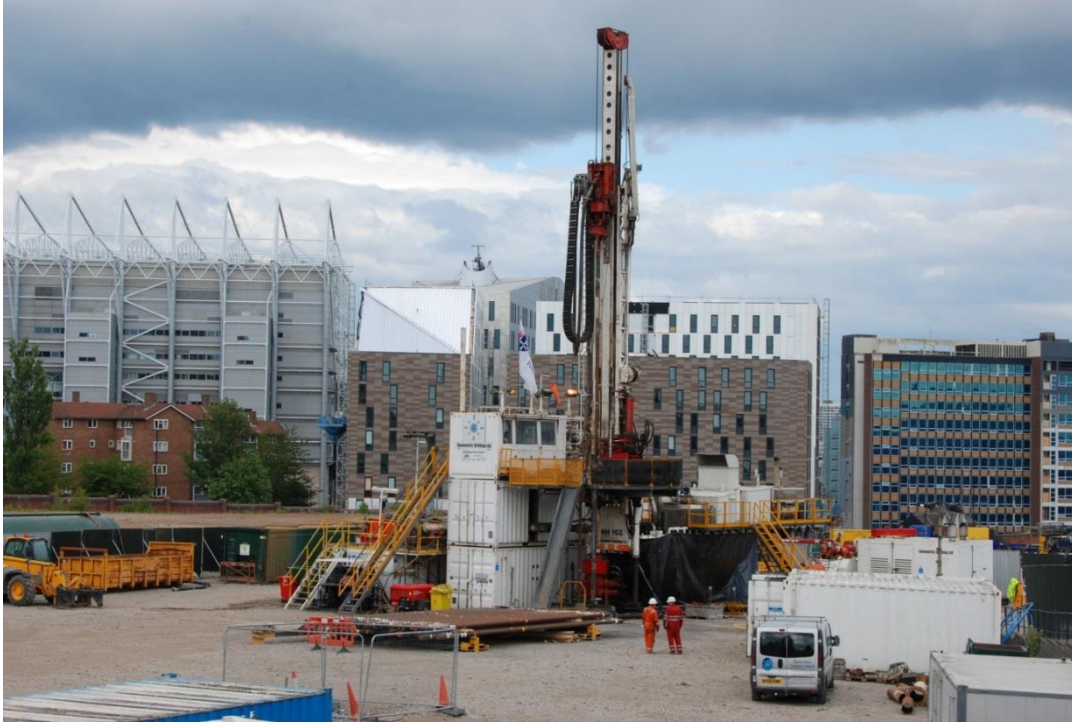
Figure 21.1 Drilling of the Science Central Borehole in the centre of Newcastle-upon-Tyne. (Credit BGS)
