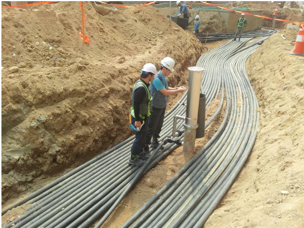
Figure 5.3b Pipe installation for a large-scale (2,100 kW) ground-source heat pump system for heating and cooling supply (see Figure 5.3a) for 1-2 zone of the new government building complex in Sejong-City, Korea.. (Photo courtesy of T-EN)
