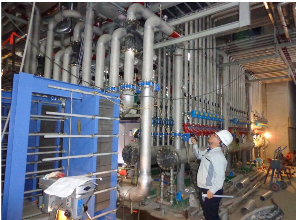
Figure 5.3a A large-scale (2,100 kW) ground-source heat pump system installation for heating and cooling supply for 1-2 zone of the new government building complex in Sejong-City, Korea. (Photo courtesy of T-EN)
