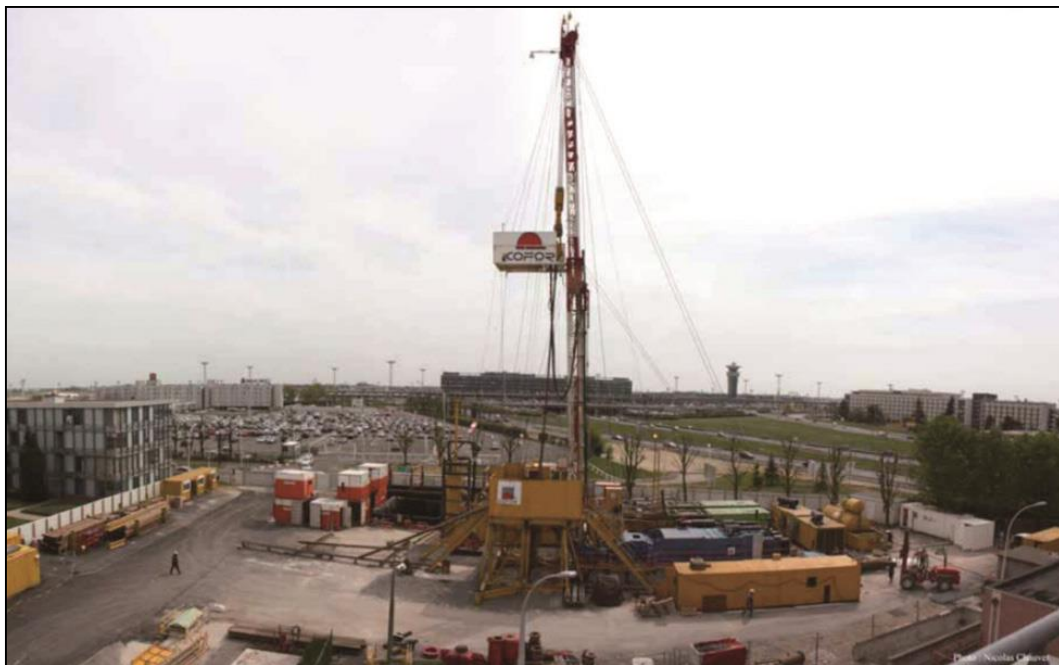
Figure 5.2 Drilling for the new geothermal heating plant for Orly Airport in Paris, France (Figure 5.1). (Photo courtesy of Romain Vernier)
