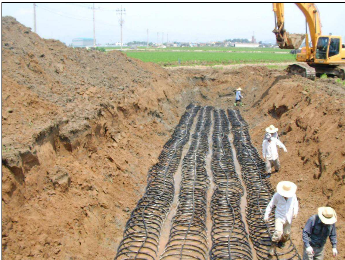
Figure 13.2 An example of geothermal heat pump system for greenhouse. (a) Installtion of slinky-type horizontal heat exchanger. (Photos courtesy Turbo Energy Co., Ltd.)
