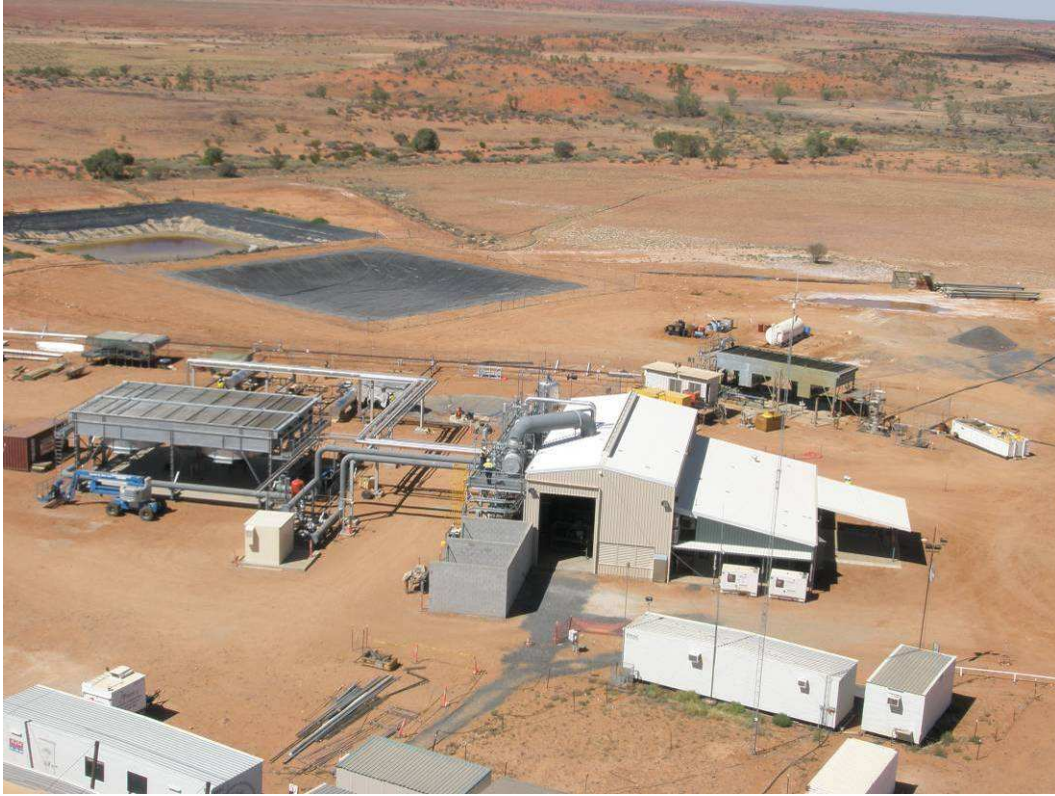
Figure 20.3 1 megawatt power station at Habanero (see turbine in Figure 20.4).
