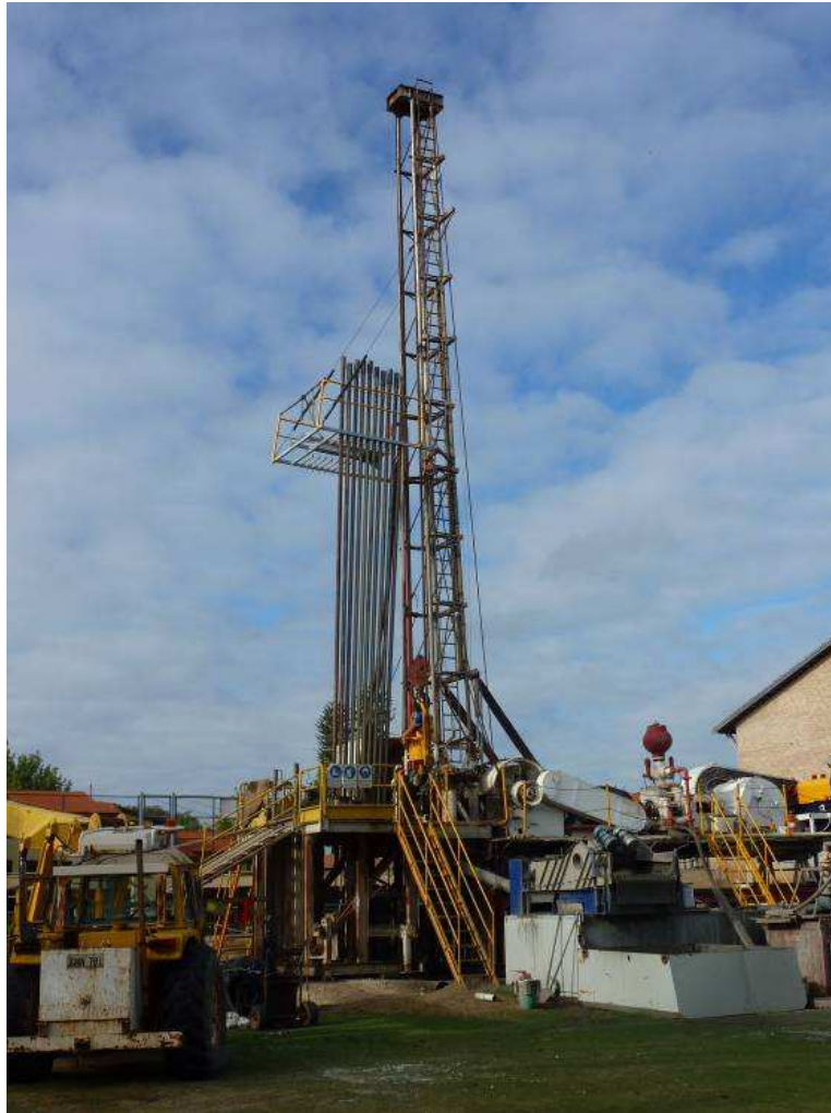
Figure 22.1 Drilling to 1000 m to heat pool in Perth.
