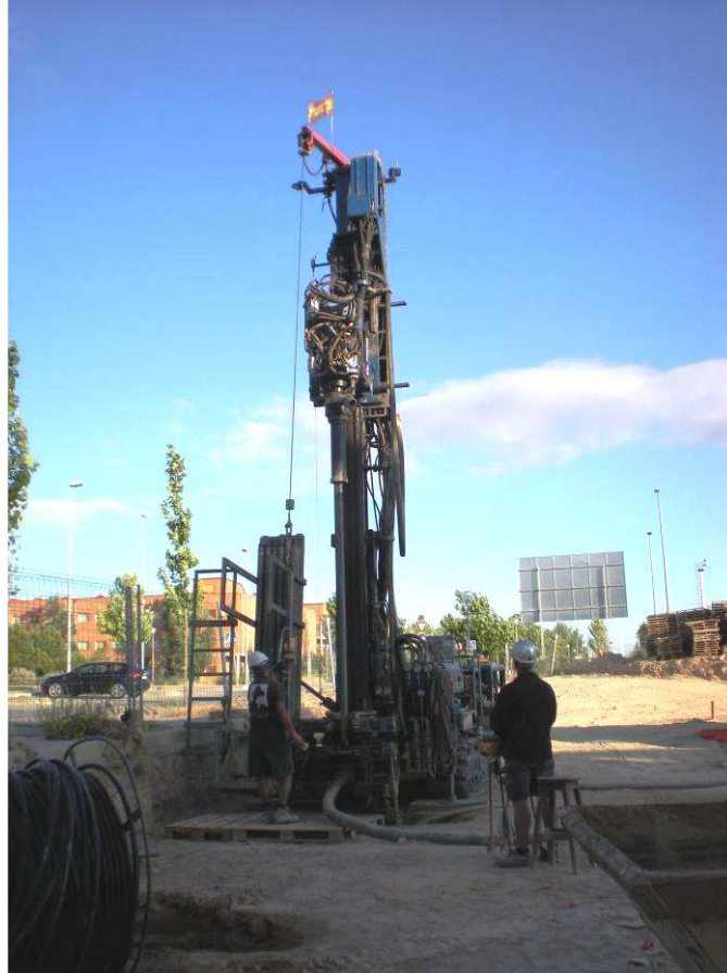
Figure I6.1 Drilling for Geothermal Heat Pump University of Alcalá de Henares. (Geoter 2010)
