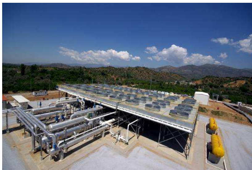
Figure 23.5 The Dora 2 Geothermal Power Plants, in Salavatli, Turkey; Ormat supplied the generating unit and technical assistance for Dora I and 2, while Mege built, commissioned and operate the two units. Dora I, 7.35 MW, was built in 2006, while Dora 2, 11.2 MW, was built in 2009. (Photo courtesy of Ormat Technologies)
