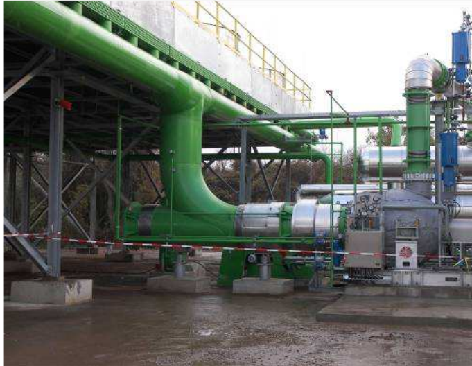
Figure 23.8 The 3.2 MW Landau Geothermal Power Plant is the first commercial plant in Germany, and the first implementation of EGS technology in an injection well. (Photo courtesy of Ormat Technologies)
