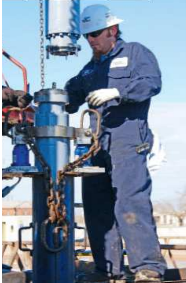
Baker Hughes INTEQ GmbH installing a pump. (Photo from: BMU, 2009a, p. 58)
