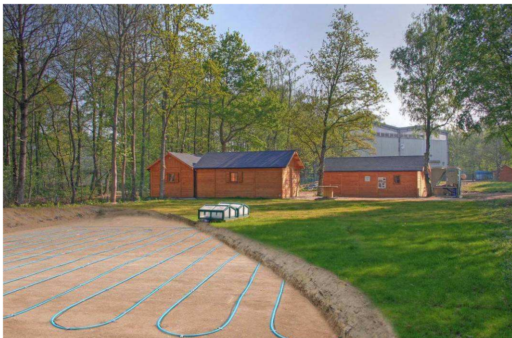
Figure 8.3 Experimental platform on GBDHP underground heat exchangers, BRGM, Orleans. (Photo courtesy of BRGM)
