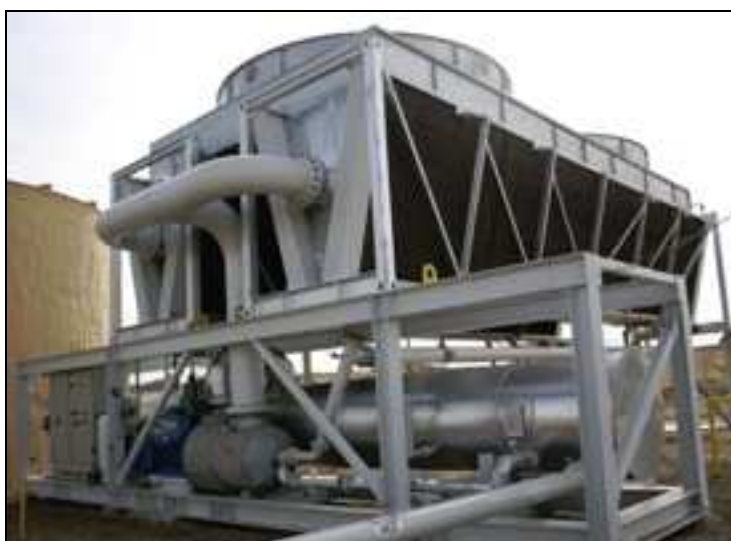
Figure 18.2 Ormat's OEC producing power from co-produced fluids in Wyoming. (Source: DOE Office of Fossil Energy)
