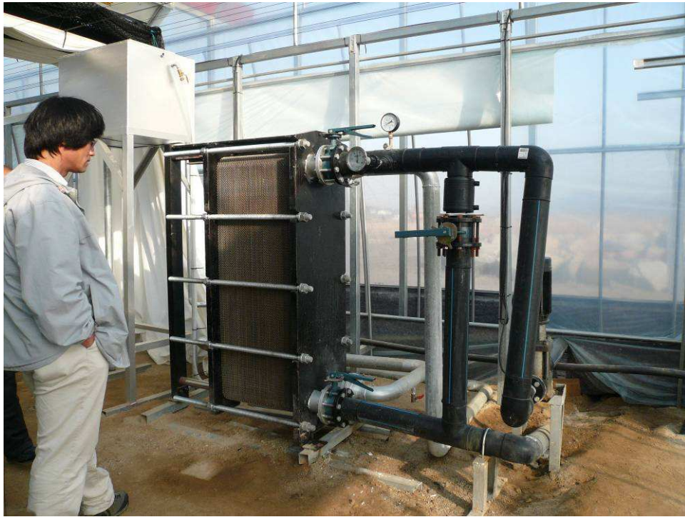
Figure 13.1c Plate heat exchanger for use of geothermal water.
