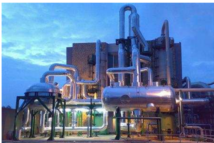
Figure 10.3 The AMIS plant for the Hg and H 2 S abatement installed at the 20 MW Nuova Gabbro power plant. (Photo courtesy Cuido Cappetti, ENEL)
