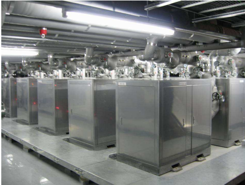
Figure 13.2b Sixty geothermal heat pumps heat and cool a large university building.
