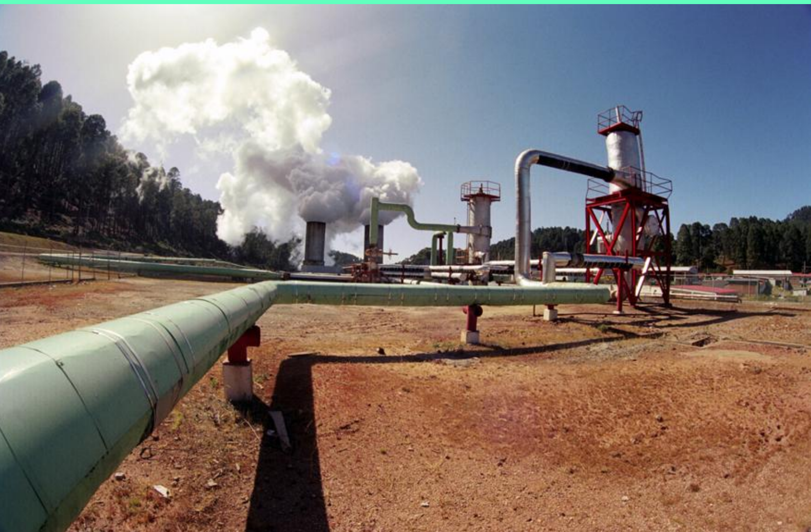
Los Azufres Geothermal Field, Mexico, showing production lines to separators, with dual silencers in background (courtesy of D. Nieva, IIE).
