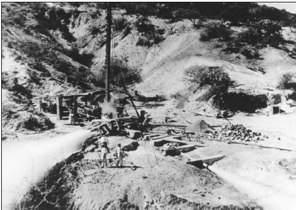
Figure 15.2 Steam flowing from the first geothermal production well drilled in 1956 at the Pathé Geothermal Field (Photo from GRC, 2003).
