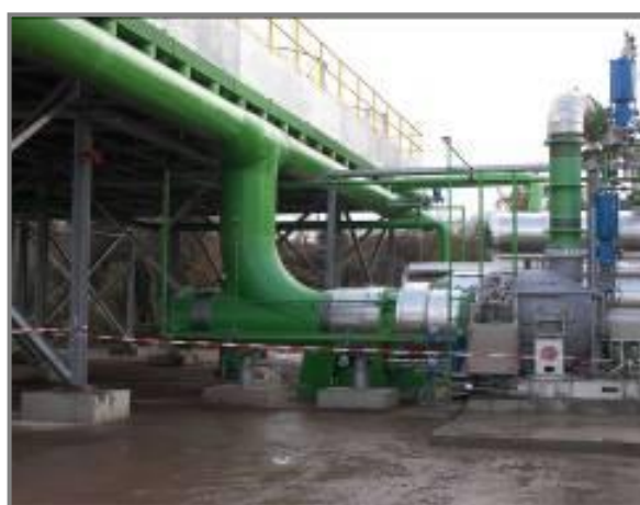
Figure 21.1 The 3.2 MW Landau Geothermal Power Plant is the first commercial plant in Germany, and the first implementation of EGS technology in an injection well (courtesy of Ormat Technologies).
