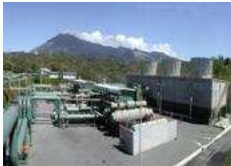
Figure 21.6 Miravalles V, Costa Rica, providing 18 MW from 166 °C brine.
