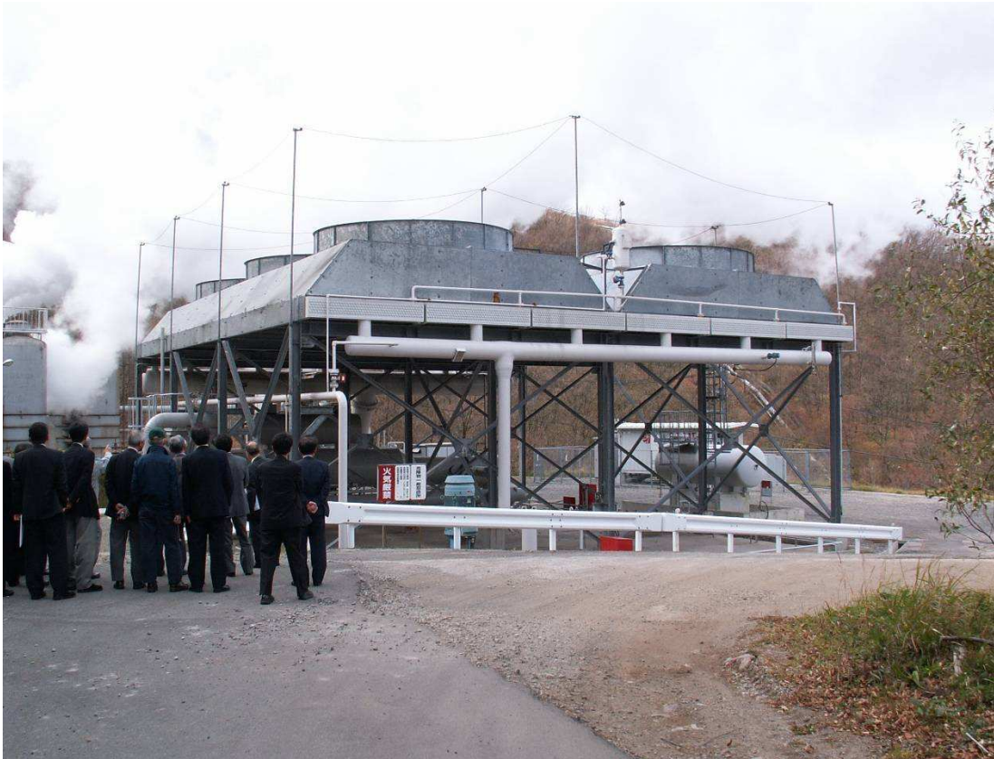
Figure 13.5 A 2000 kW demonstration binary power plant in the Hatchobaru geothermal power plant. Observers are from Ten'ei-mura. (Photo taken 9 November 2004).
