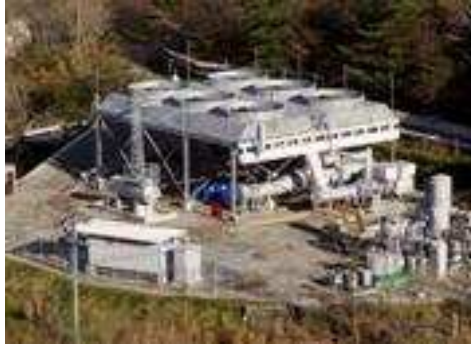
Figure 21.5 Hatchobaru, Japan providing 2 MW from a 143°C brine.
