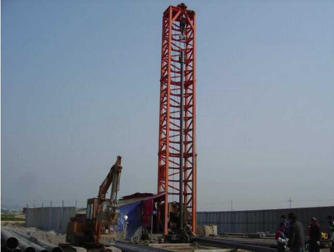
Figure 14.2 Drill rig for the production well, BH-4, Pohang geothermal project.
