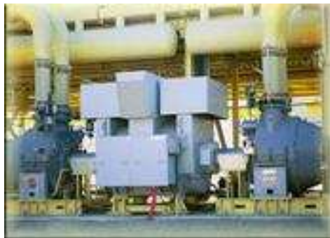
Figure 21.7 Brady, Hot Springs, USA, providing 6.5 MW from 110 °C brine.
