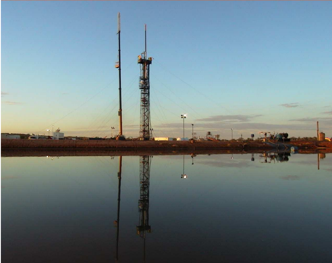
Figure 19.4 Snubbing unit setup over Habanero 2, 20 March 2006. The actual snubbing unit was set 33 m above ground level on a scaffold and 10,000 psi rated 7-inch riser pipe.
