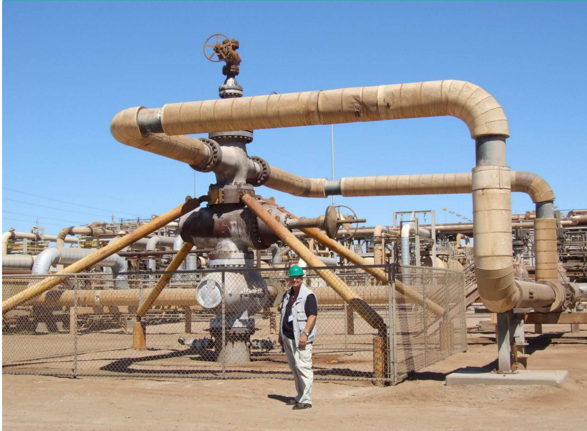
50 MW e well at Salton Sea Geothermal Field, Imperial Valley, California, USA with scientist posing for scale (photograph courtesy of M.A. Mongillo).
