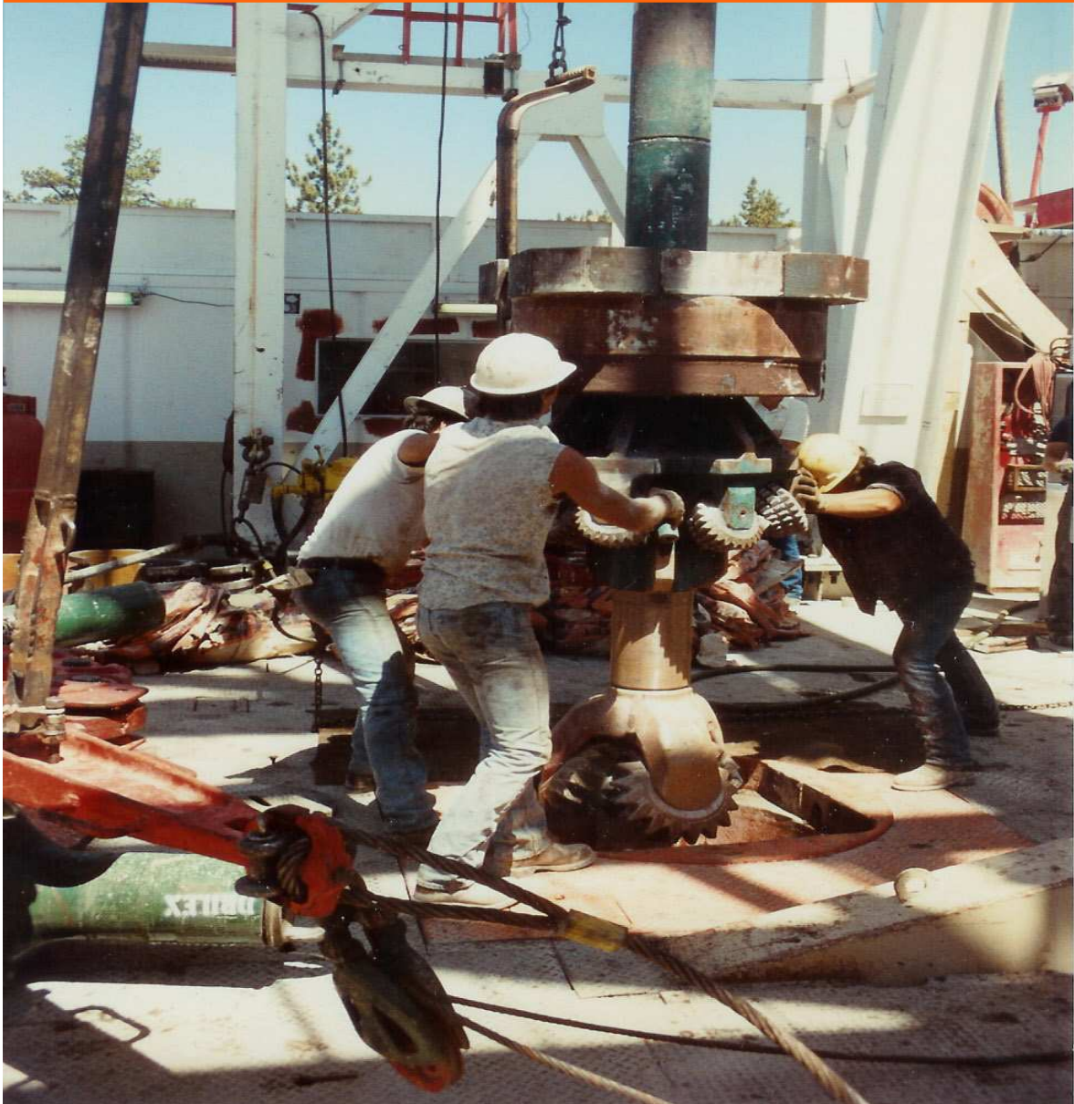
Drilling the Magma Energy exploratory well in 1989 at Long Valley, California, USA, showing the 26-inch bit with the 36-inch hole-opener above it (courtesy of John Finger).
