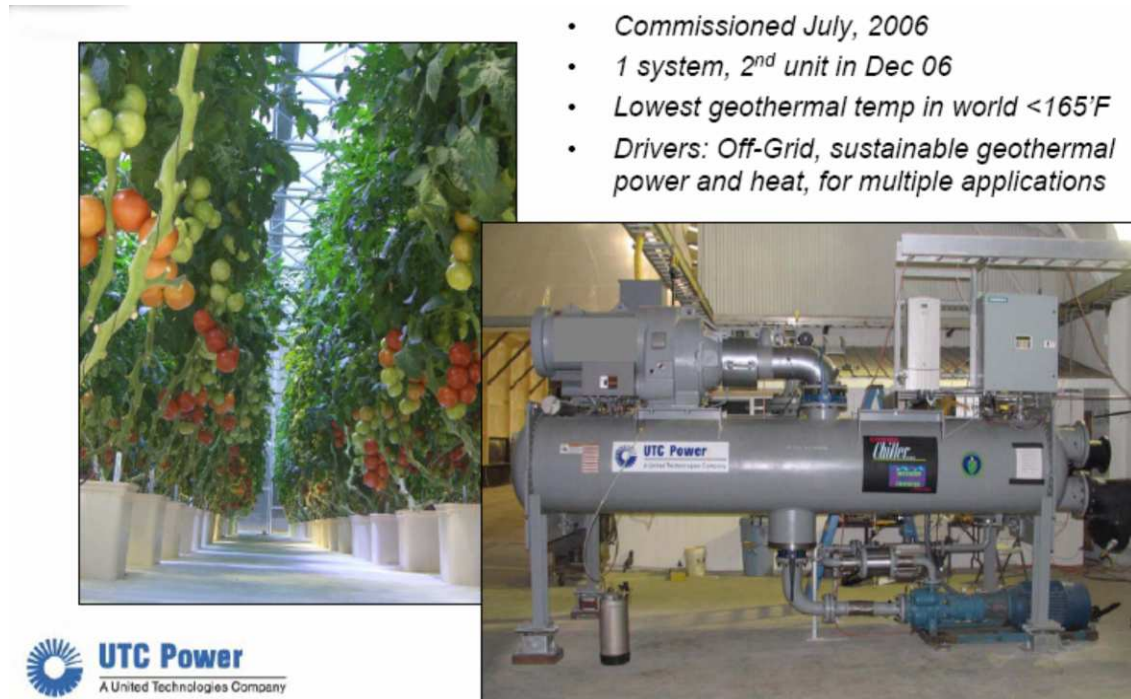
Figure 18.1 Unit 1 of Chena Power Plant (UTC Power).
