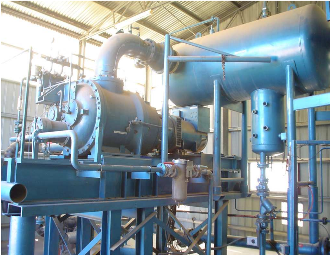
Figure 8.5 Organic Rankine Cycle Turbine and Oil Separator, Birdsville, Queensland. Courtesy of Ergon Energy
