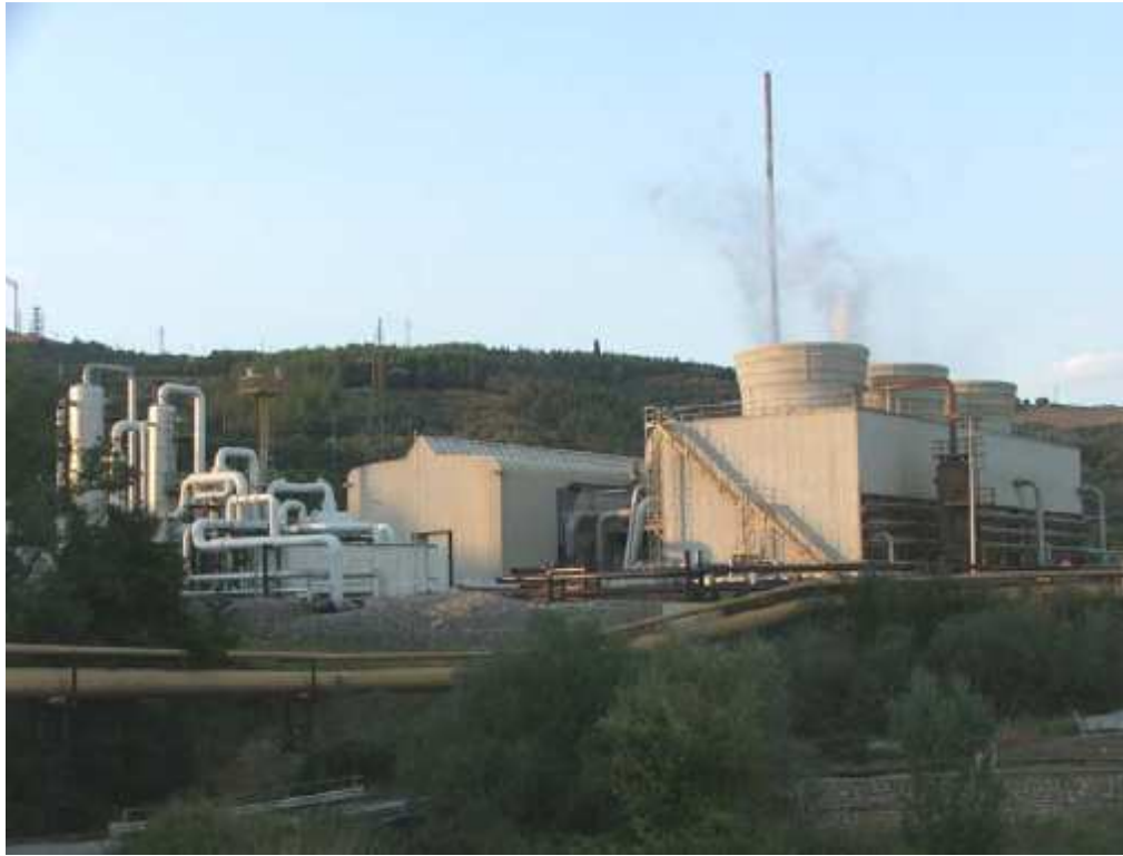
Figure 12.2 A 20 MW e unit with the AMIS hydrogen sulphide and mercury emissions abatement system at the left.
