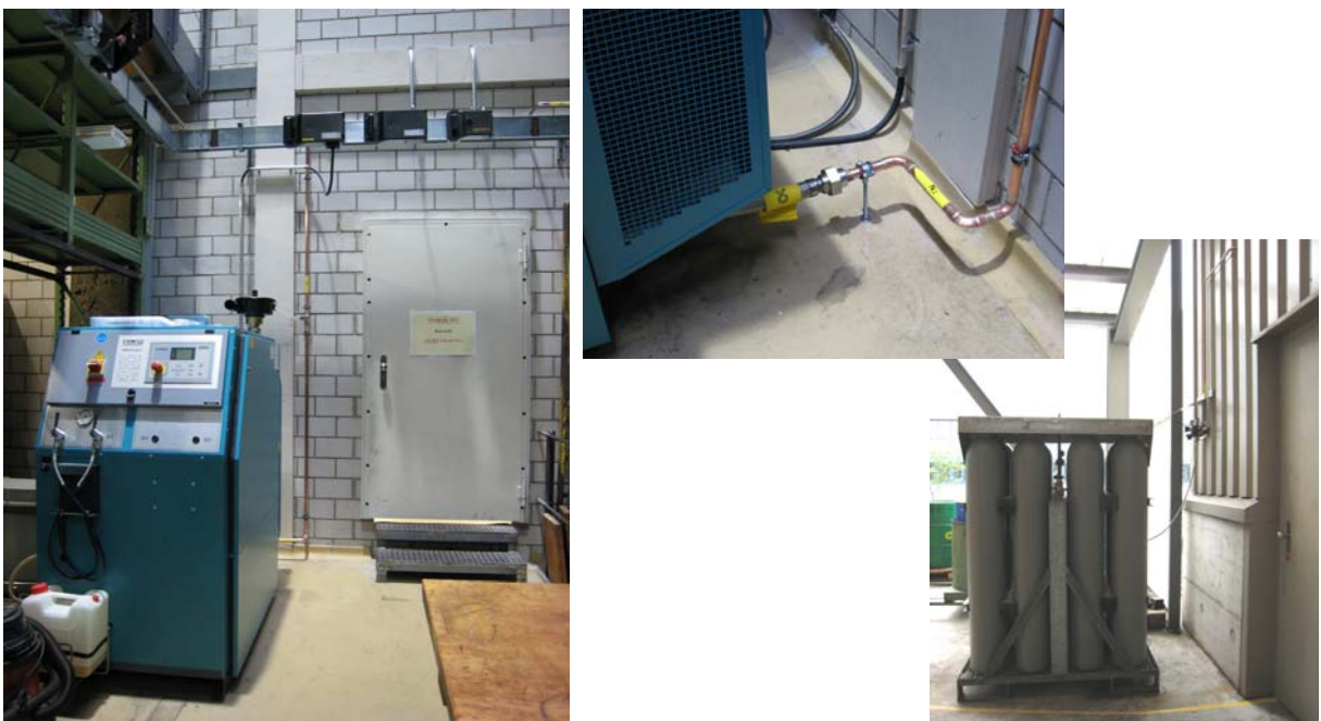
Figure 3: Compressor with dual (air-N 2 ) operation capability.
