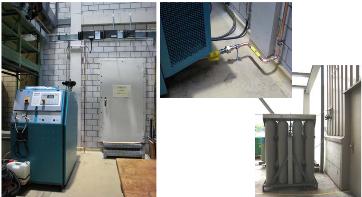
Figure 3: Compressor with dual (air-N 2 ) operation capability.
