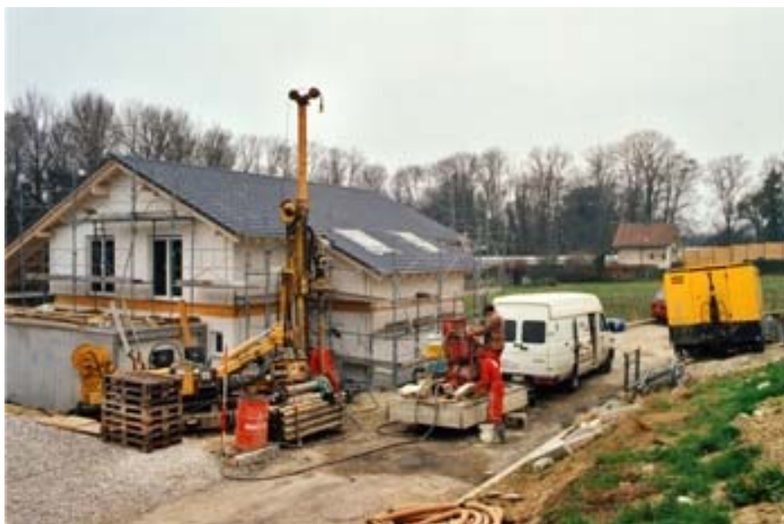
Figure 17.1 Construction site where a BHE-type geothermal heat pump system is being installed at Bevaix/NE, Switzerland.
