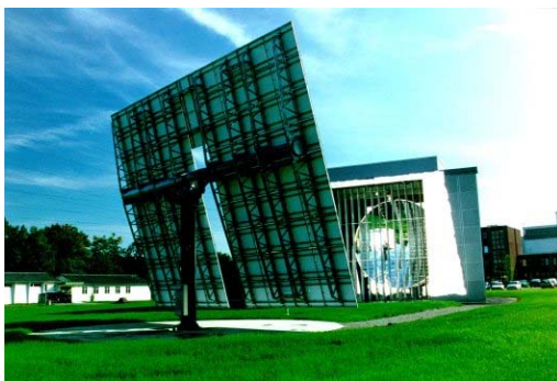
Figure 3: PSI's High-Flux Solar Furnace (HFSF) consists of a 120 m 2 sun-tracking flat heliostat on-axis with an 8.5 m diameter paraboloidal concentrator [19]. It delivers up to 40 kW at peak concentration ratios exceeding 5000 suns (1 sun = 1 kW/m 2 ). The solar flux intensity can be further augmented to up to 10,000 suns by using CPC secondary concentrators. A Venetian blind type shutter located between the heliostat and the concentrator controls the power input to the reactor. http://solar.web.psi.ch/
