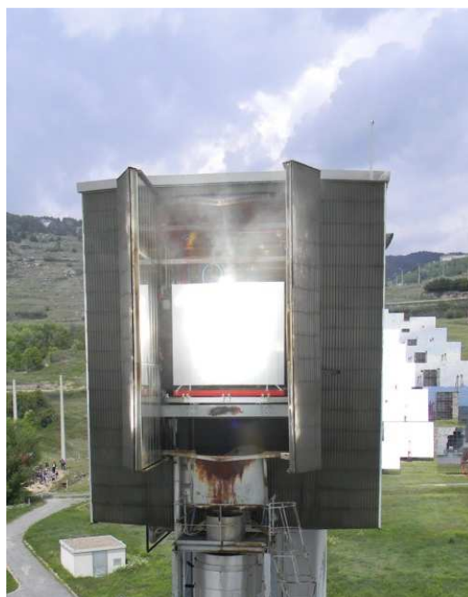
Figure 11: Heliostat field with central heliostats tracking the sun (left); doors of the MWSF tower partly open showing spilled radiation on the radiation shield (right).
