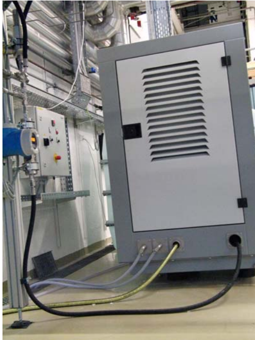
(a) The high pressure pump of the cooling water 2 network.
