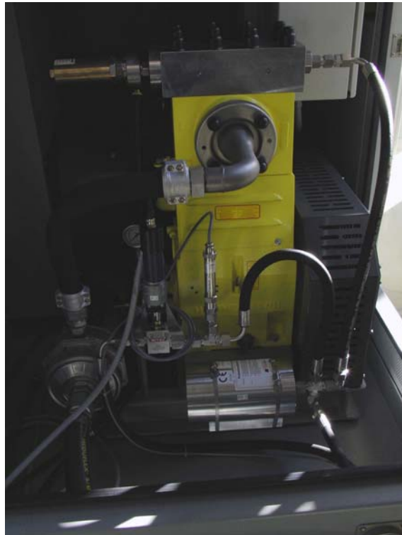
Figure 5.9: The high pressure pump of the cooling water 1&3 network.
