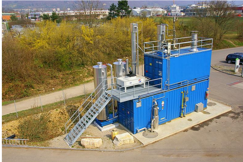
Fig. 3.2 Installation for biogas purification using glycol washing at the biogas plant in Pratteln (Source: Keller, Biopower Nordwestschweiz AG)
