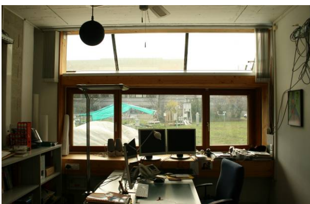
EC glazings in the clear configuration (Tv=50%, SHGC=38%)
