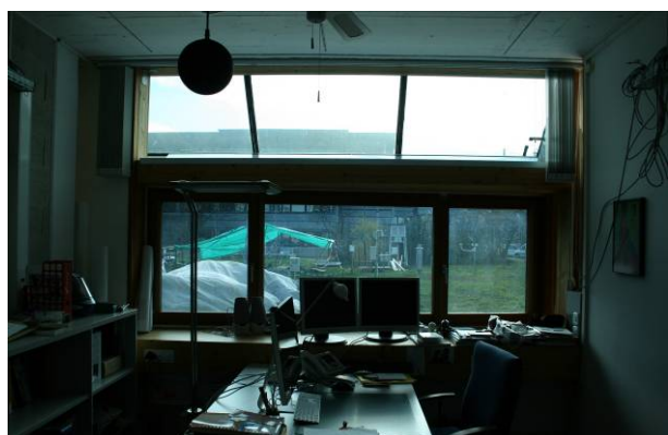
EC glazings in the dark configuration (Tv=15%, SHGC=12%)
