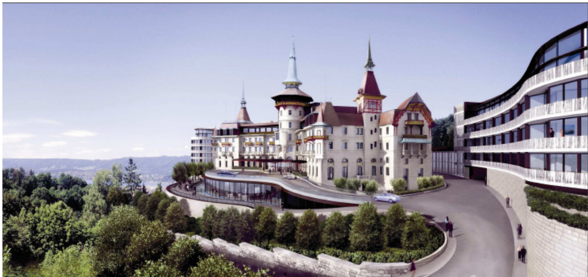
Figur 1: Das neue "The Dolder Grand".
