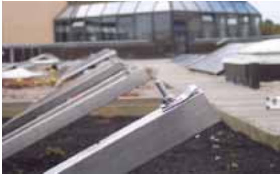
Fig. 3: The module can be hung into the bracket Fig. 4: Craft brackets are pushed in at the bottom
