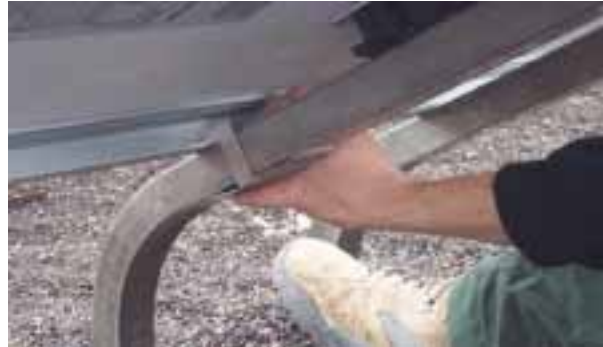
Fig. 3: The module can be hung into the bracket Fig. 4: Craft brackets are pushed in at the bottom
