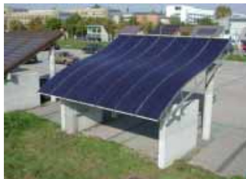
Fig. 4: Freestyle photovoltaic roof (Demosite), (source: LESO / EPFL)
