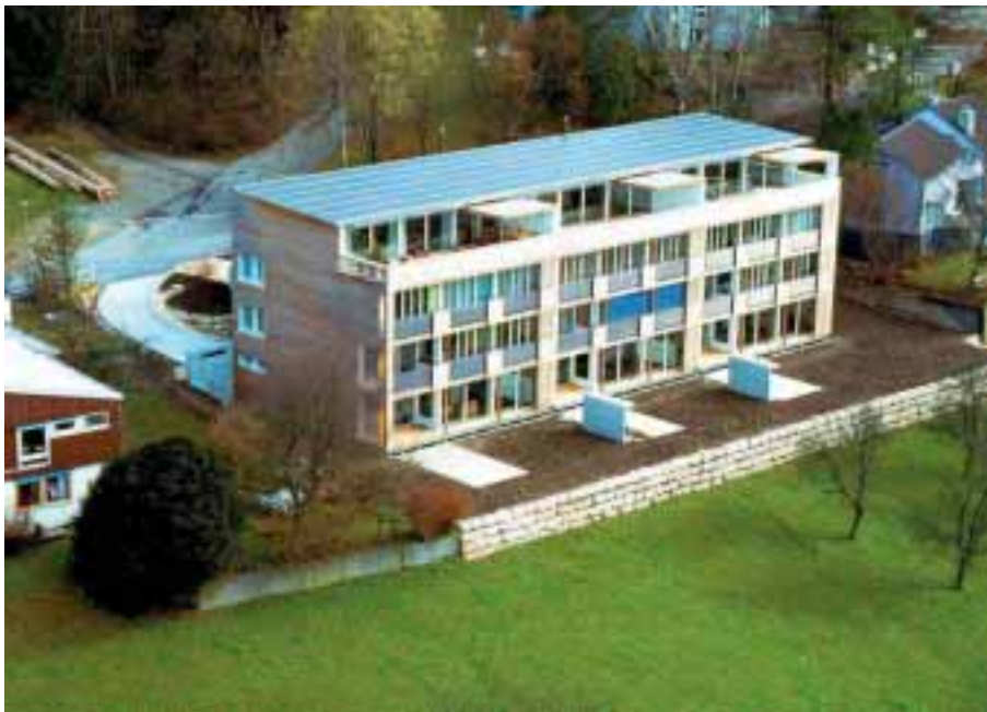
Fig. 9: 'Sunny Woods' PV installation with amorphous triple cells, (source: Kämpfen Architects)
