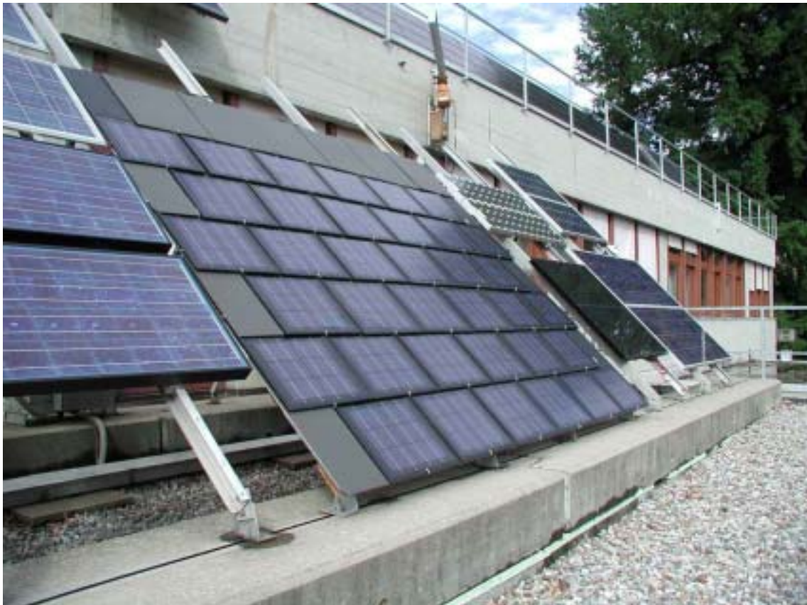
The Figure 2 shows the test site at LEEE and the new PV roof shingle from the side. As can be seen on the foto, the shingles are 100% plan and identical in size such as a normal conventional fibre cement roof shingles. Identical is also the entire roofing system, and even the mounting procedure, so that roofers do not require extensive special training.
