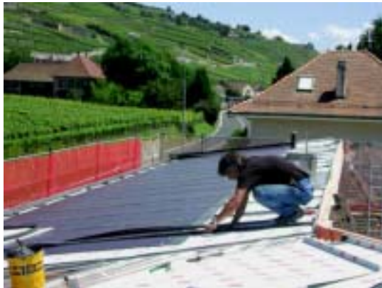
Fig. 11: Mounting of the PV roof integrated Freestyle® installation with amorphous triple cells in Lutry (Photo: Solstis)
