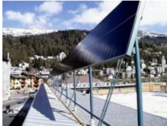
Fig. 16: 16.8 kWp installation with CIS cells St. Moritz (Photo: LEEE-TISO)
