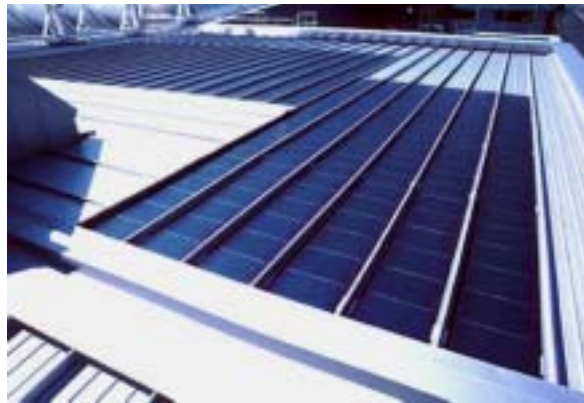
Fig. 19: 3 kWp PV Eurodach amorph Flums (Photo: NET AG)
