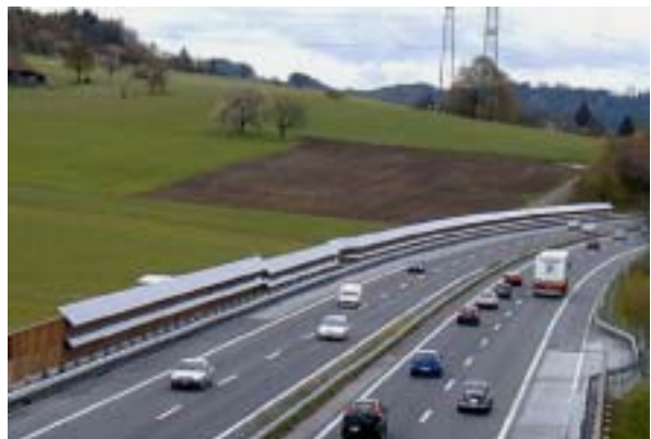
Fig. 20: 75 kWp noise barrier installation A1 Safenwil (Photo: BFE)
