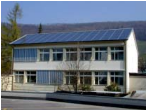
Fig. 15: 12.75 kWp roof integration Wettingen (Photo: NET AG)
