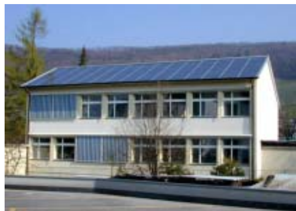
Figur 31: 12.75 kWp Dachintegration Wettingen (Bildquelle NET)
