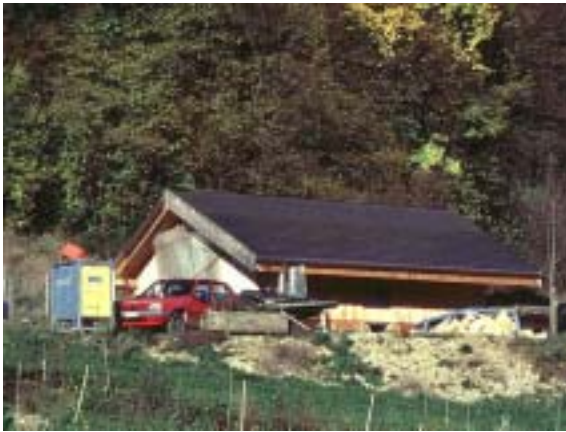
Figur 20: Autonome 3 kWp Dachintegration in Soyhières (Bildquelle NET)
