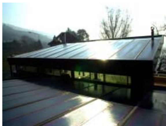
Figur 25: Dachintegration Freestyle® in Lutry (Bildquelle Solstis)
