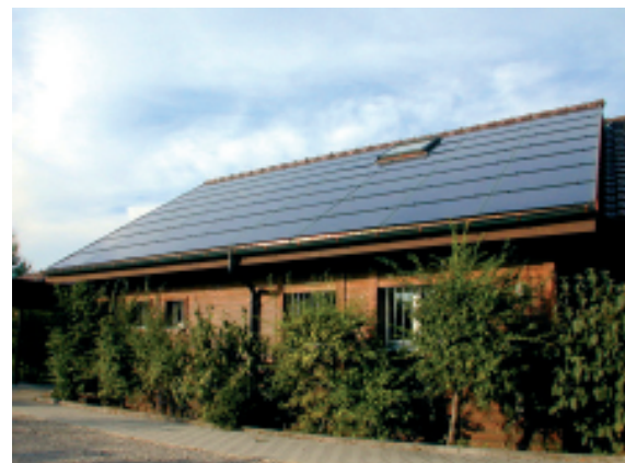
Figur 22: 15 kWp Dachintegration Weiermatt (Bildquelle NET)
