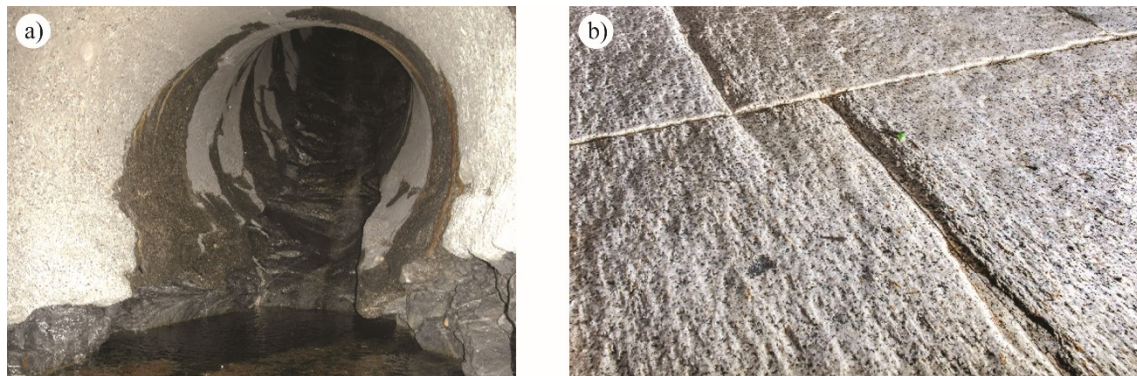
Figure 1: Hydroabrasion examples: a) deep abrasion into the concrete invert and rock underground at the Val d'Ambra SBT (photo: M. Müller-Hagmann), b) hydroabrasive damages at the granite lining of the Pfaffensprung SBT (photo: VAW) (adapted from Mueller-Hagmann 2017)
