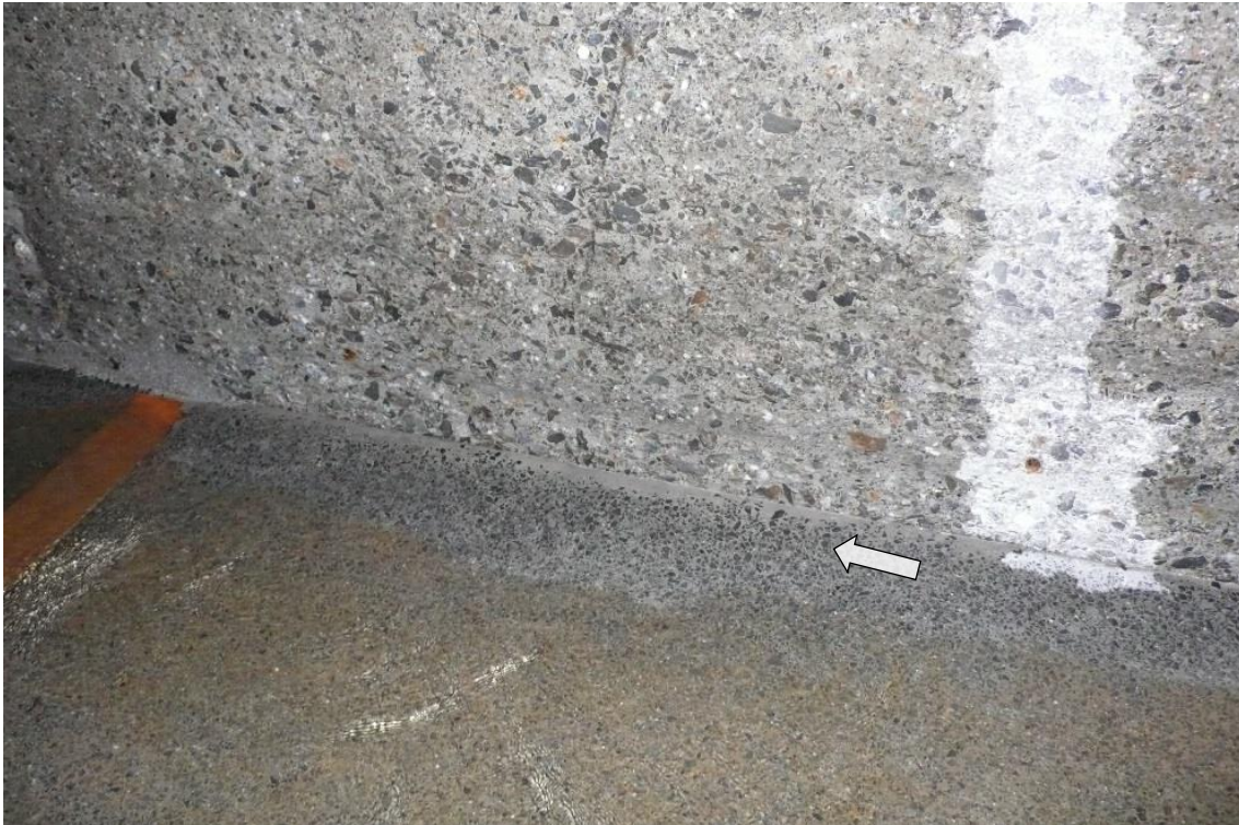
Figure 16: Minor damage due to abrasion in the PC test field and at the lower part of the wall (normal concrete), picture taken 2012
