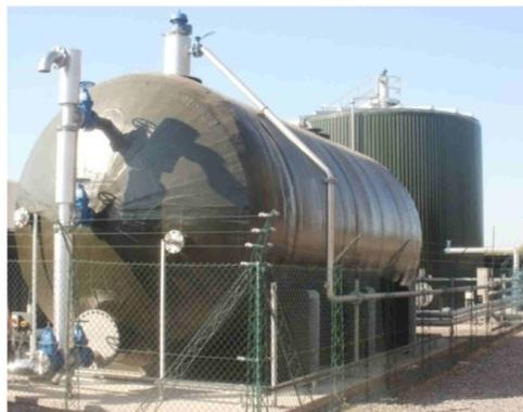
**Figure 4-7 :** Digesteur "Plug and Play" de Marches Biogas. [Source: Marches Biogas]
