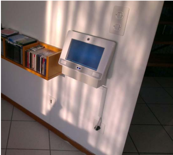
Figure 33: Remote PC unit installation
